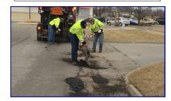
**What Is A Pothole?** While several factors contribute to the creation of potholes, they are distresses in the pavement that can create a failure of the pavement. This failure causes the pavement material to crumble and create a void in the pavement.
