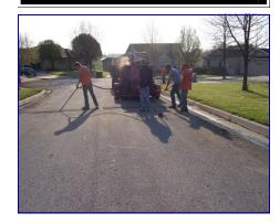
What Is Crack Sealing? A key preventative maintenance technique where small cracks are filled with a rubberized asphalt product creating thick "snake like" lines on the street. Sealing the cracks helps prevent water from getting into the street payement and causing potholes.
