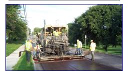
What Is Microsurfacing? Microsurfacing is a preventative street sealing technique that uses a pre-mixed slurry of rock, polymer asphalt binders, cement, and filler materials to seal the entire roadway at a depth of about 3/8th of an inch. It is applied over the top of the pavement.
