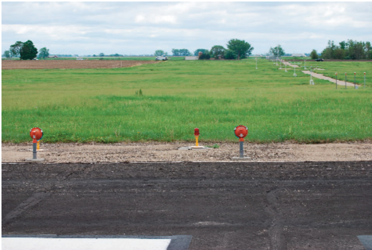
Photo 67: View south, east edge of Runway 15/33, toward Hwy 40.
