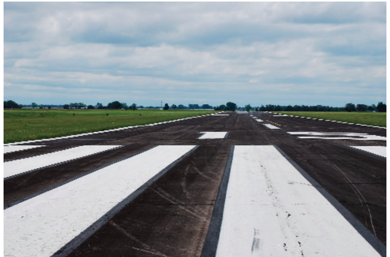
Photo 46: View south on Runway 15/33.
