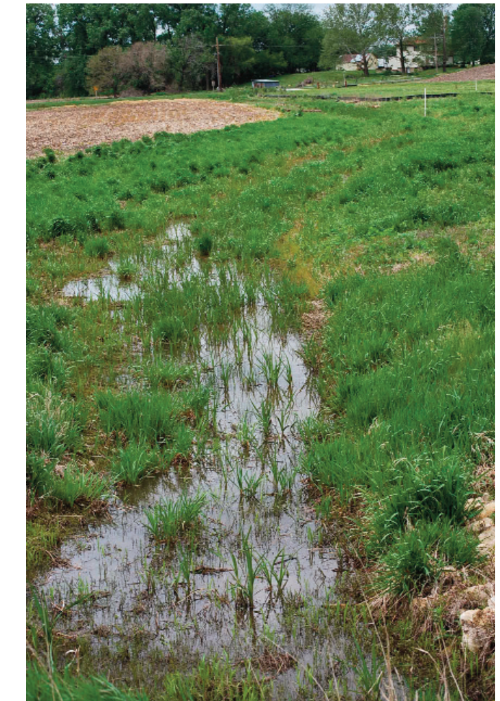
Photo 112: View west off Airport Road culvert span showing water volume after heavy running through property toward Hwy 40. This area was noted as avian habitat in 2012 WHA.
