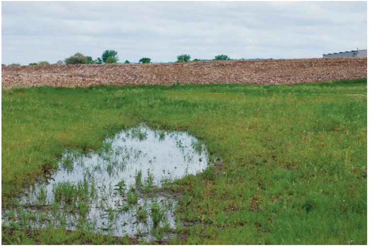
Photo 7: Looking North from airport septic system pump station off Hwy 40.
