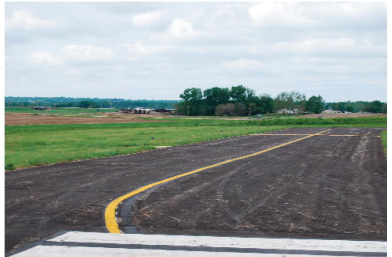
Photo 71: View south, west edge of Runway 15/33, toward Hwy 40.
