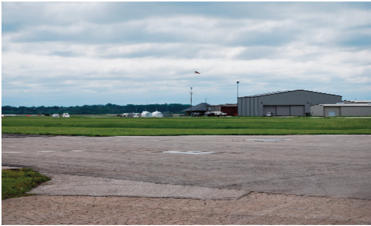
Photo 21: View southeast from KU hangar apron on west side of airfield.
