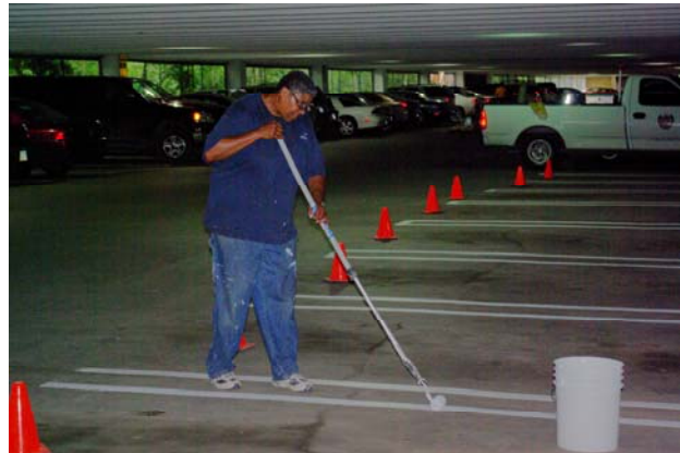
Parking garage re-striping
