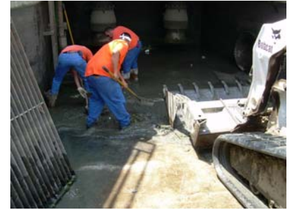
North Lawrence pump station Clean out
