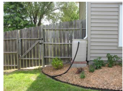
Rain barrel made at workshop
