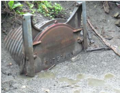
Kansas River levee Working on re- certification
