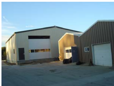
New tire shop, in progress
