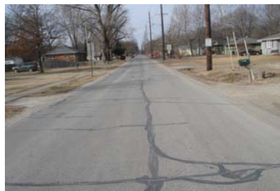
Crack-seal treatment
