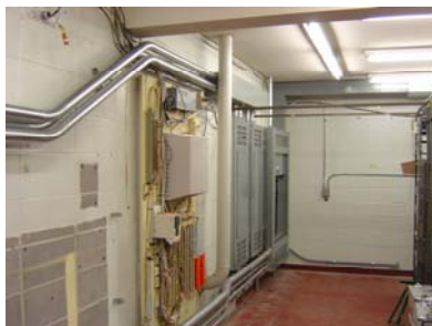
Parts room electrical project
