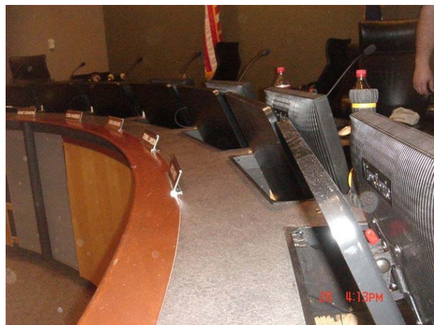
Work station installation in City Commission room
