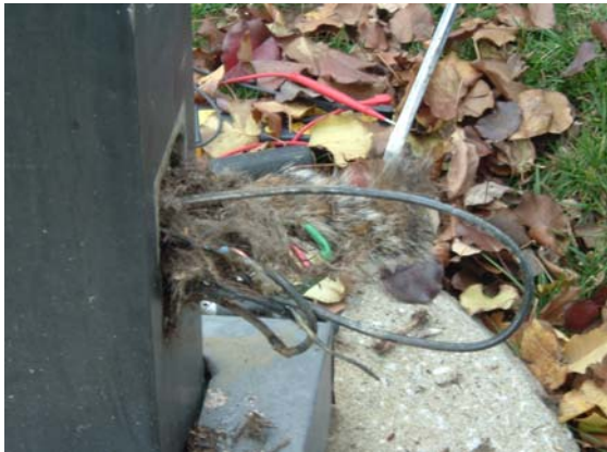
Trouble-shooting electrical problem at ITC
