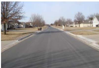
Trail Road, curb & gutter, mill & overlay
