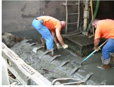
North Lawrence pump station Clean out
