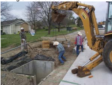
Catch basin construction
