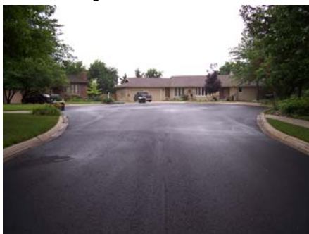
Mill and overlay
