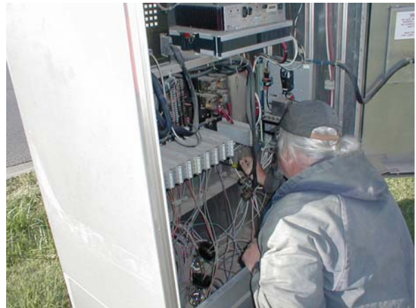
Final wiring inspection, 15 & Iowa
