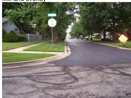
Mill and overlay
