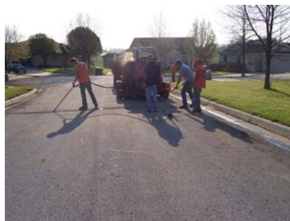
Mill and overlay
