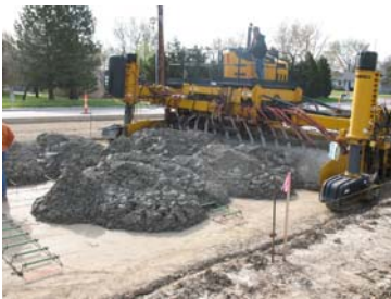
Paving on west side of road
