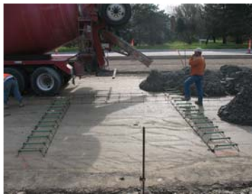
Paving on west side of road
