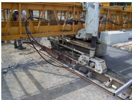
Paving in progress
