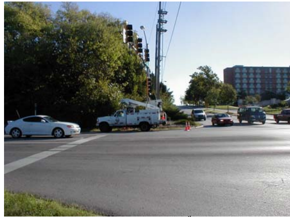
Wiring right turn arrow at 15 th and Iowa
