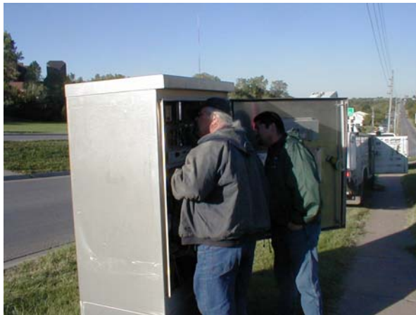
Signal controller re-wiring
