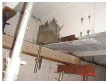
Expansion joint and beam repairs
