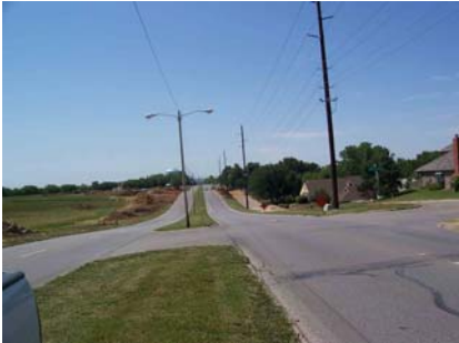
Kasold Drive, prior to reconstruction
