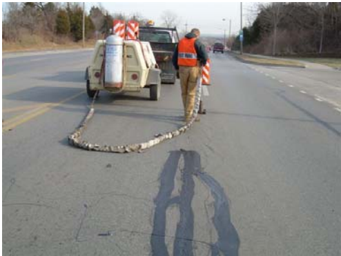
Crack sealing, 6 th Street
