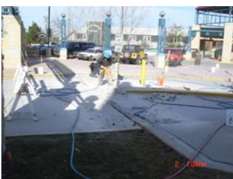
Expansion joint and beam repairs
