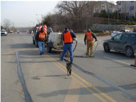
Crack sealing, 6 th Street
