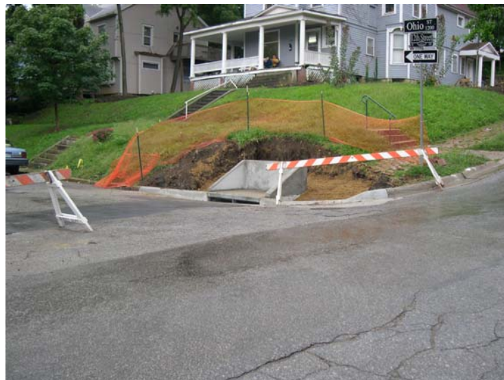
Reconstruction of curb inlets and storm sewers, 12 th and Ohio
