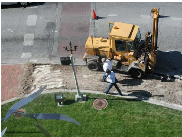
Reconstruction of pedestrian crossing outside City Hall
