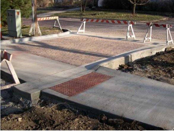
Alley reconstructed after sewer replacement, 8 th and Maine
