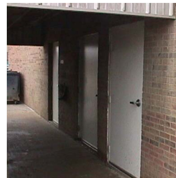
New walk-in doors, north side.
