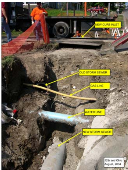
Reconstruction of curb inlets and storm sewers, 12 th and Ohio
