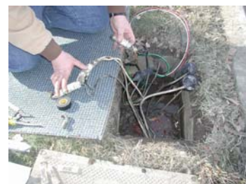
Bill Musick, Electrician, trouble-shoots downtown lighting issues.
