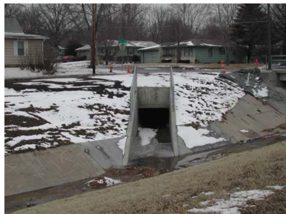
System outlet after construction
