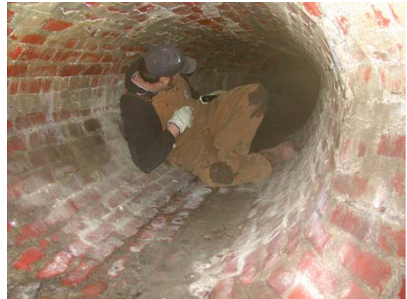
Inspecting a collapsed storm sewer near 7 th and Maine
