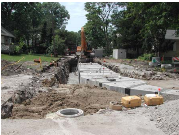
Storm and sanitary sewers under construction
