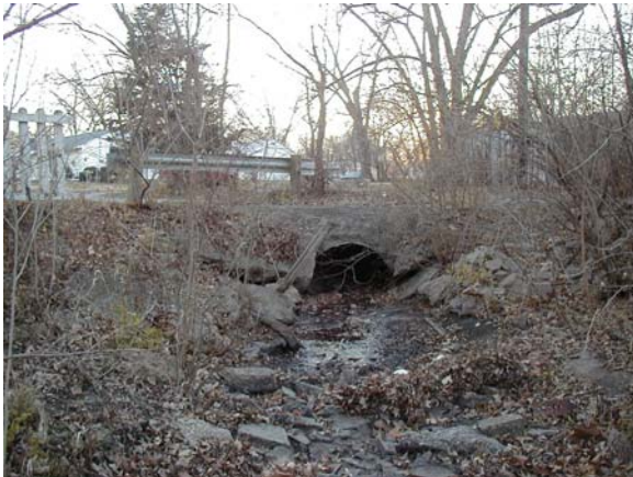
System outlet before construction
