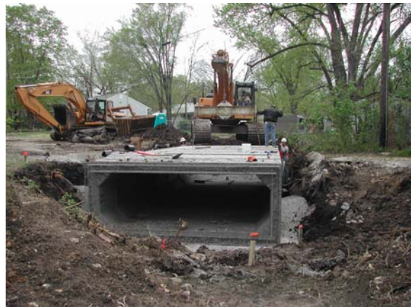
System outlet during construction
