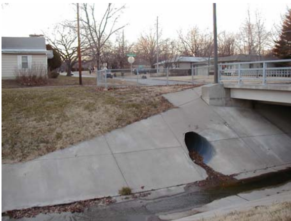
System outlet before construction
