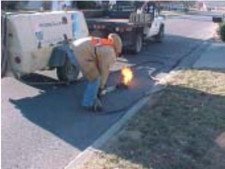
City workers crack-sealing on Lawrence Avenue
