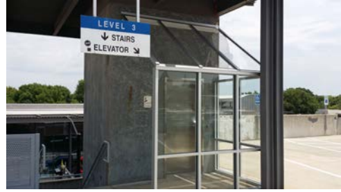
Elevator enclosure New Hampshire garage
