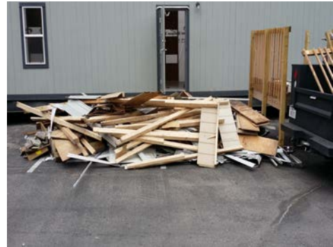
Clean up from Library temporary offices
