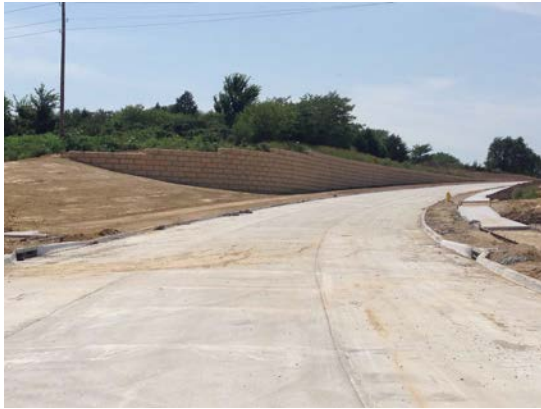
Venture Park infrastructure
