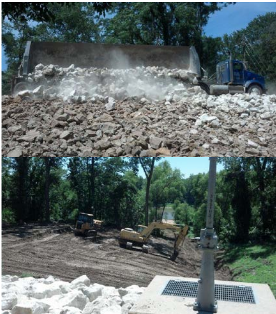
Work on Kansas River Levee
