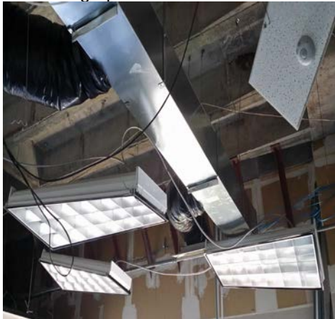
City Hall 4 th floor remodel
