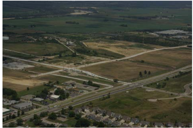
Venture Park infrastructure
