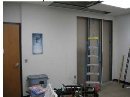
Door removed at Health Building
