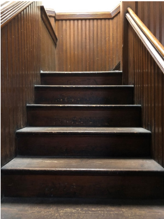
Figure 10: Staircase, northwest tower
