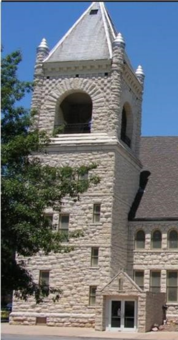
Figure 13: Entry and stairwell to old fellowship hall
