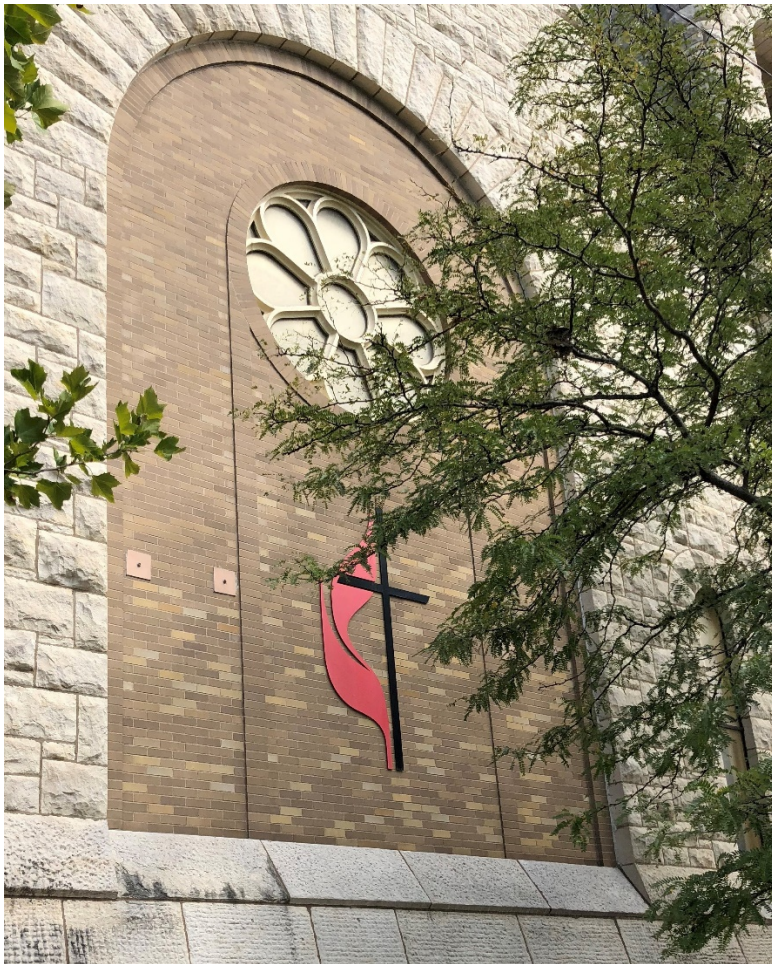
Figure 6: Former arch window
