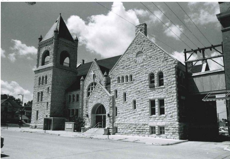
Figure 27: Bridge across alley, date unknown (between 1968 and early 1980s)
