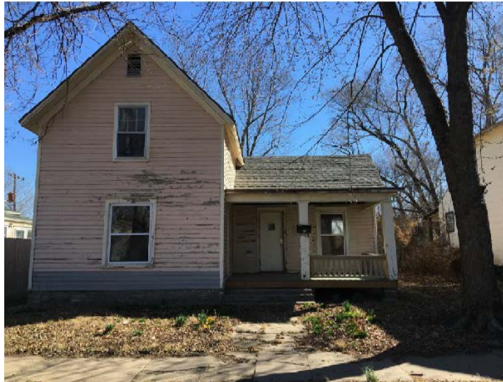
Front of the structure located at 1124 Rhode Island Street.
