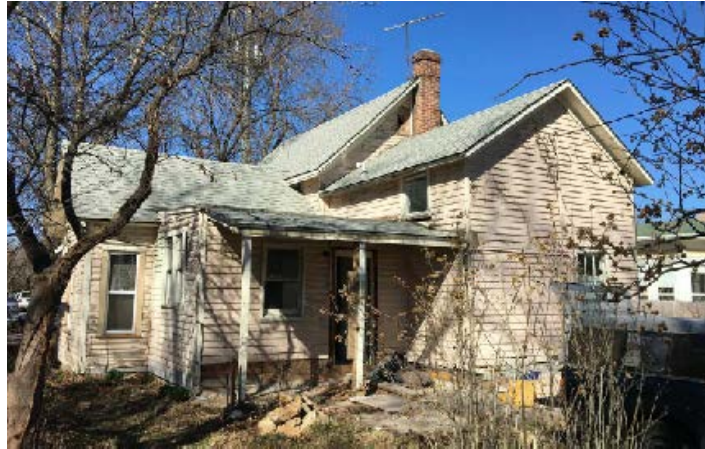
View of rear of the structure from the alley.
