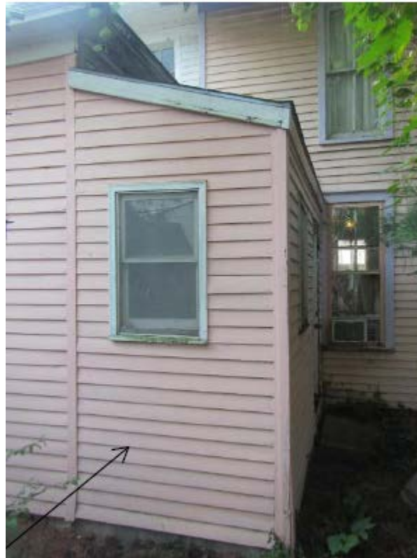
Shed to be removed
