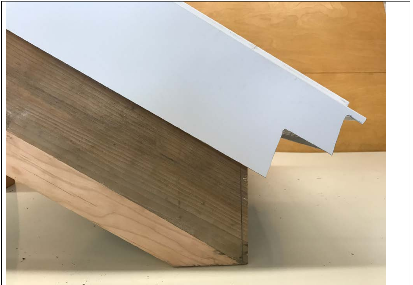
Mock-up with Rafter, Tongue and Grove, OSB, Rigid Foam Insulation, Air Space, OSB, and Metal Roof with Metal Trim
