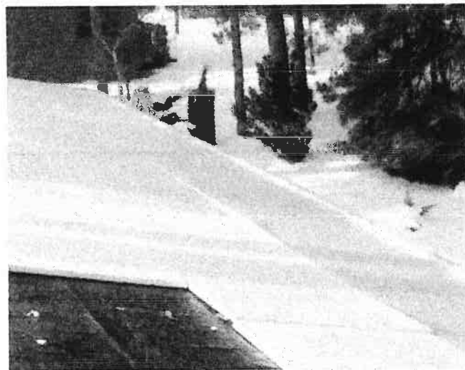
Figure 1. After installing a double 2x4 nailer around the perimeter of the roof, the crew fills in the field with a layer of 1½-inch rigid foam (above). A second layer is installed over the first, with 2x4 purlins between each row to provide nailing for the spacers to follow (right).
