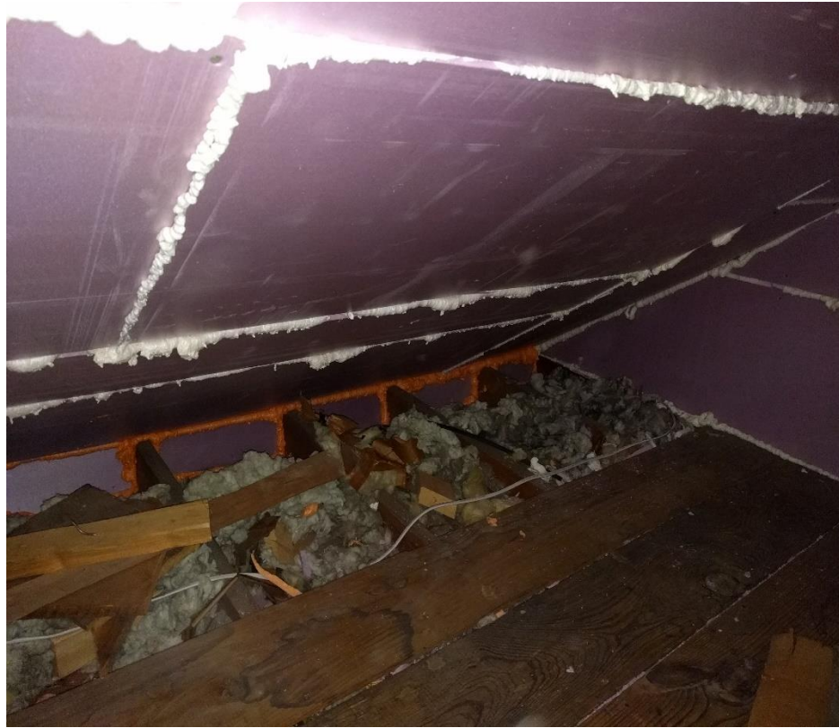
All Photos – Foam board insulation has now been installed and sealed inside of every cavity. The insulation was then sealed into place with spray foam.
