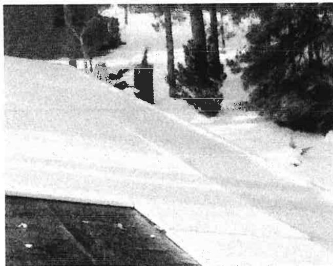
Figure 1. After installing a double 2x4 nailer around the perimeter of the roof, the crew fills in the field with a layer of 1½-inch rigid foam (above). A second layer is installed over the first, with 2x4 purlins between each row to provide nailing for the spacers to follow (right).
