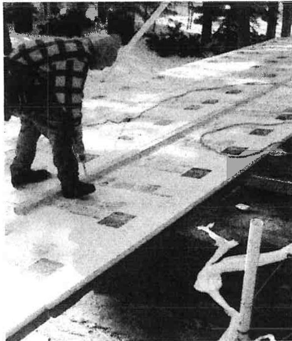
Figure 1. After installing a double 2x4 nailer around the perimeter of the roof, the crew fills in the field with a layer of 1½-inch rigid foam (above). A second layer is installed over the first, with 2x4 purlins between each row to provide nailing for the spacers to follow (right).
