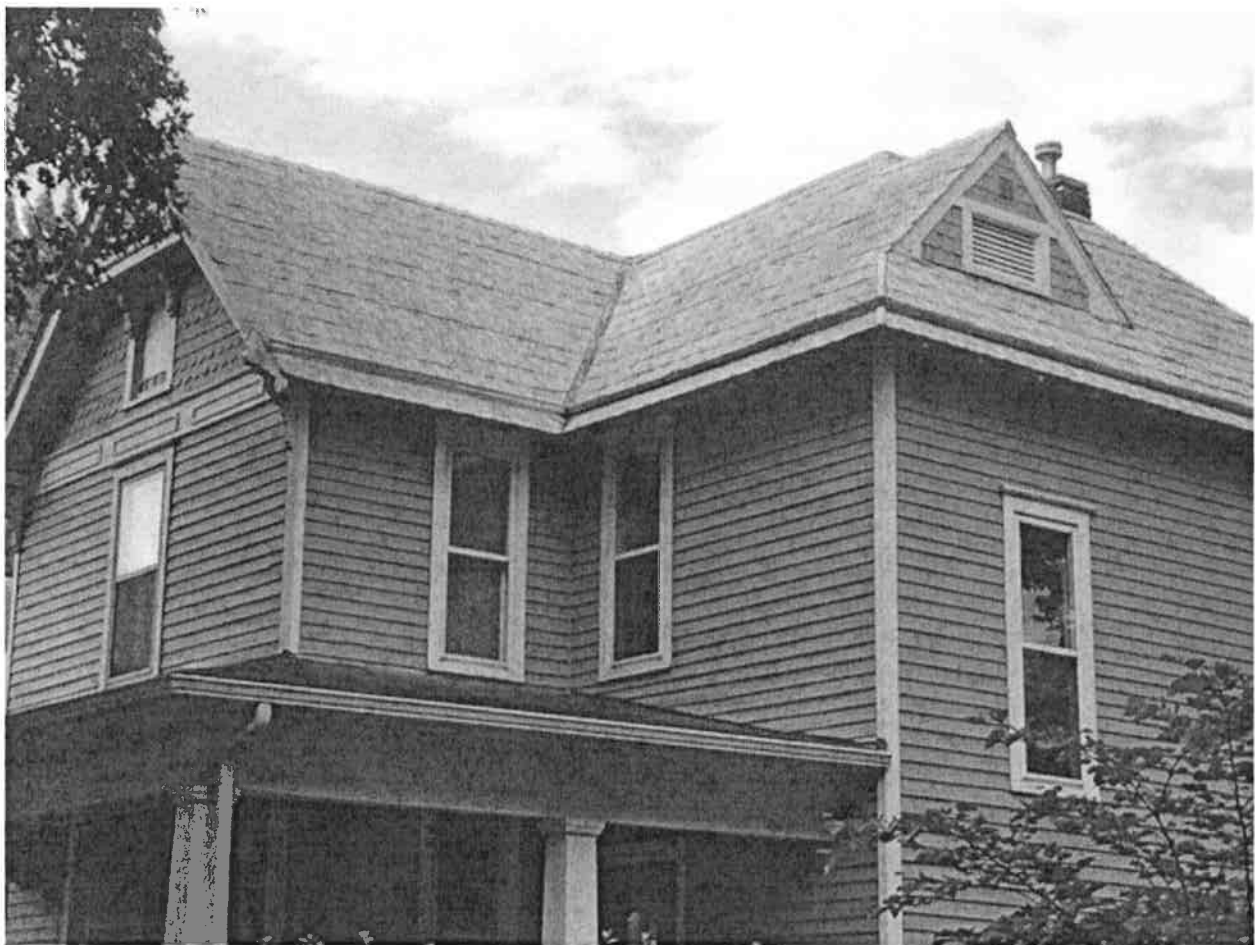
631 Ohio: Older (original?) metal shingles.
