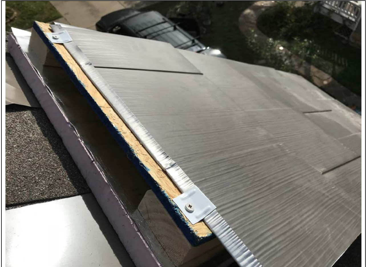
Mockup as placed on roof: existing shingle roof, rigid foam insulation, 1 ½ wood spacer, OSB, metal shingle (Applicant photo looking down to ground)
