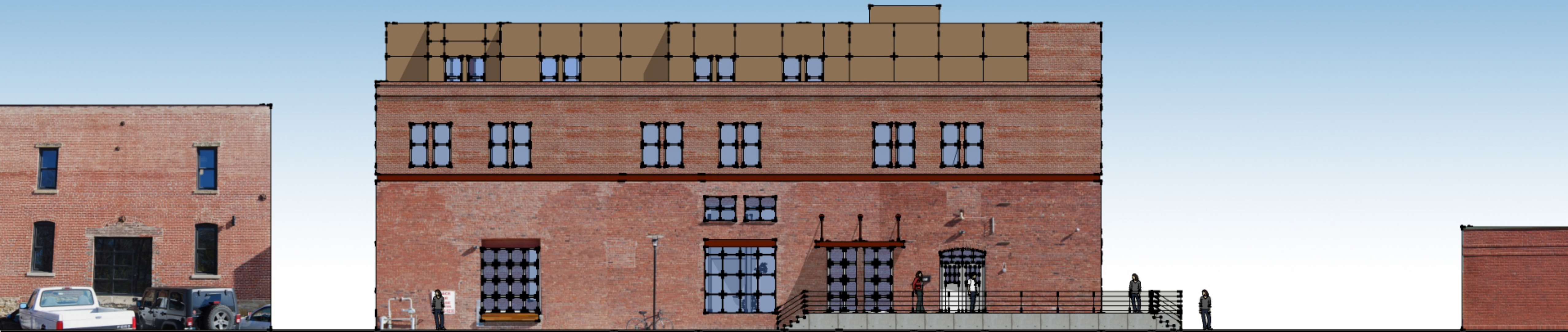
WEST ELEVATION, PENNSYLVANIA
