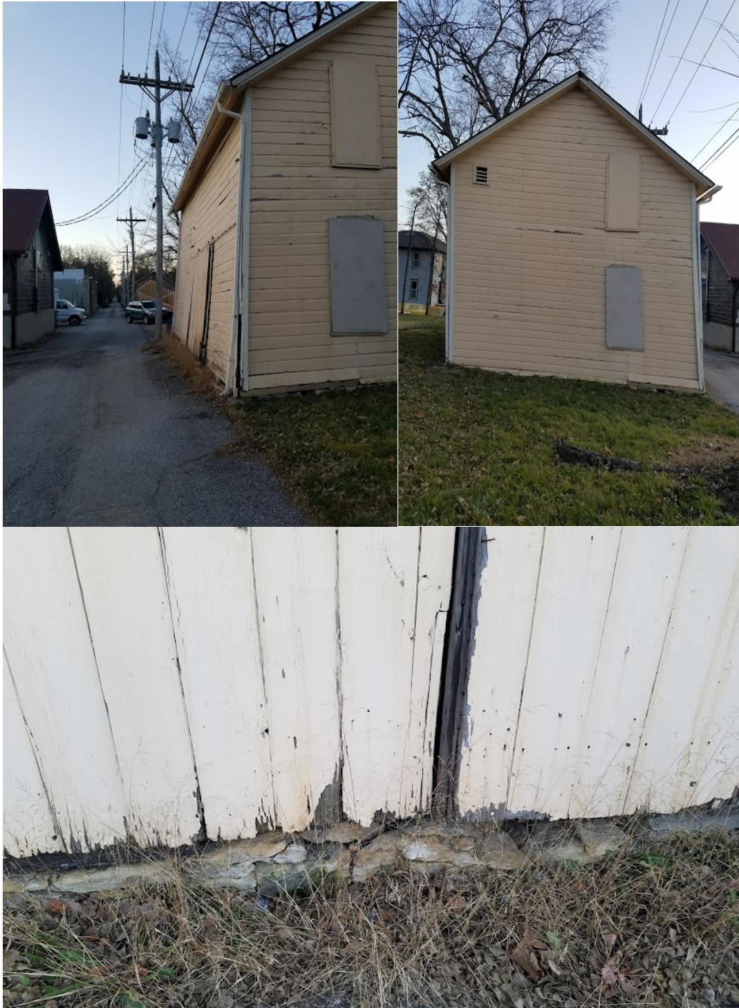
Foundation and siding in bad shape.
