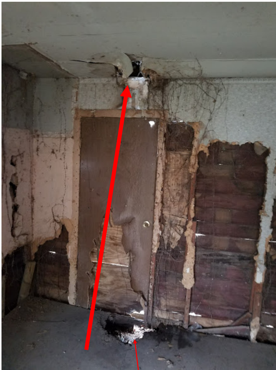
Hole in the foundation and ceiling.
