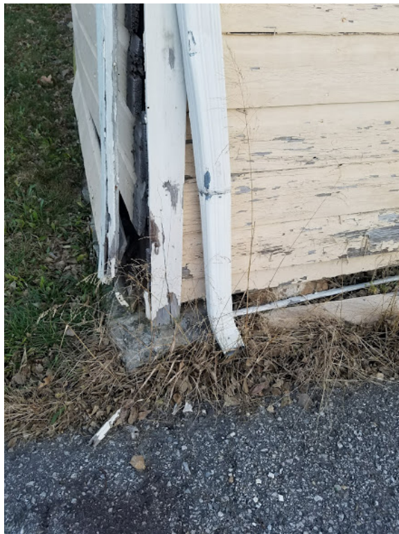
One corner of the garage is detached from the other end.
