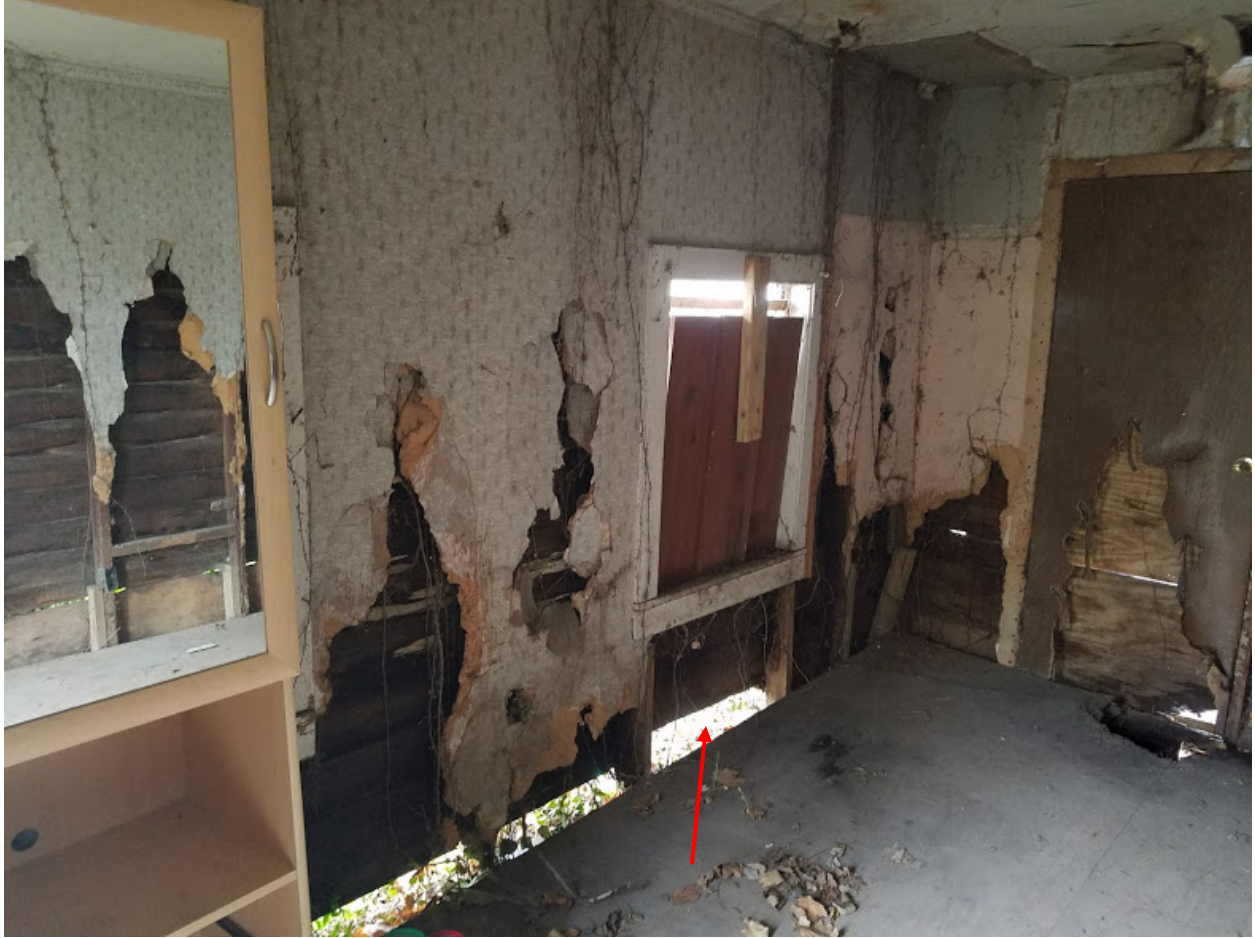
No windows but plywood to cover the holes. Foundation and siding deteriorating.
