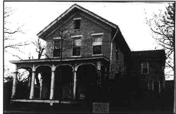
Figure 2. T.H. Eldridge House at 945 Rhode Island.
