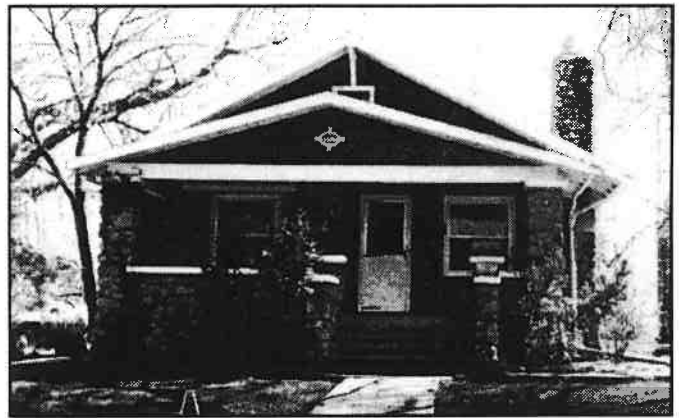
Figure 20. Craftsman bungalows, such as this one located at 1428 Pennsylvania, are noted for their use of natural materials, here rough-laid limestone and wood shingles.
