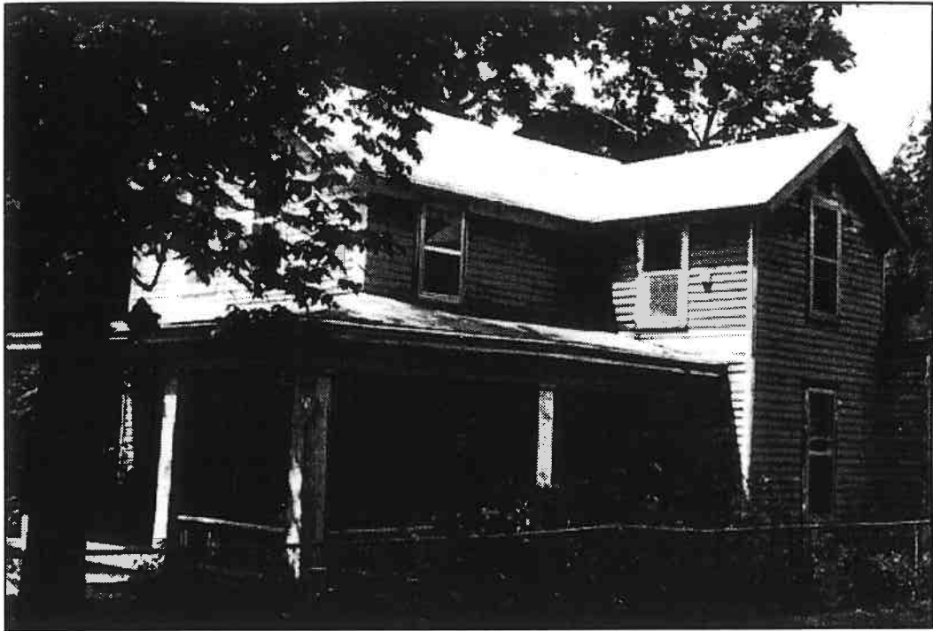
Figure 14. 1225 Delaware, a typical two-story frame example of the gable-front & wing, where in East Lawrence the larger wing is generally the gable-front portion, rather than the side wing.
