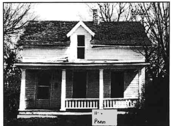
Figure 15. A variation from the typical I-house form at 1144 Pennsylvania, with an off-center door and 1 1/2 stories in height.
