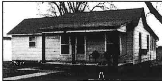
Figure 17. A former hall-&-parlor at 910 New Jersey, with additions to the side and rear, as well as siding and porch alterations.
