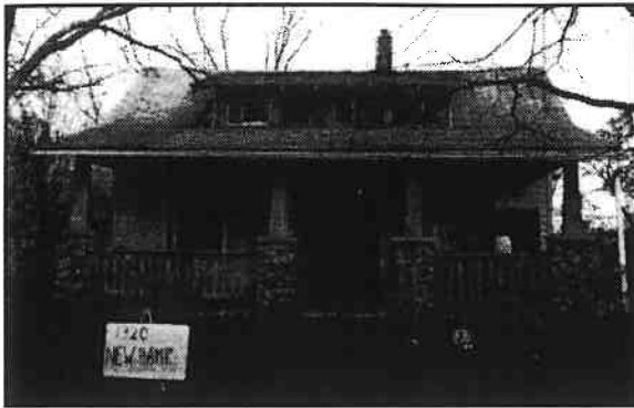
Figure 21. 1320 New Hampshire, with the typical bungalow sweeping roof extending over the porch.
