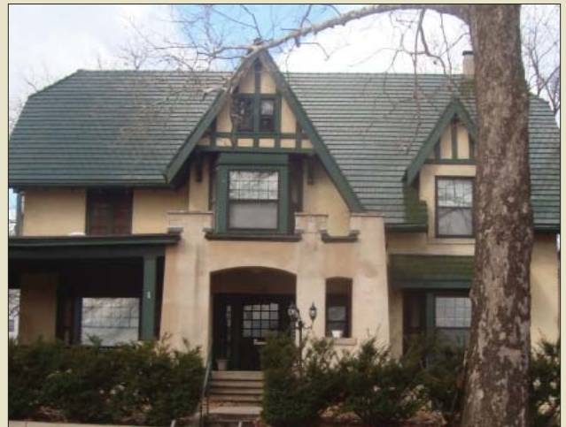
Maintain original decorative roof elements such as these cast roofing tiles.
