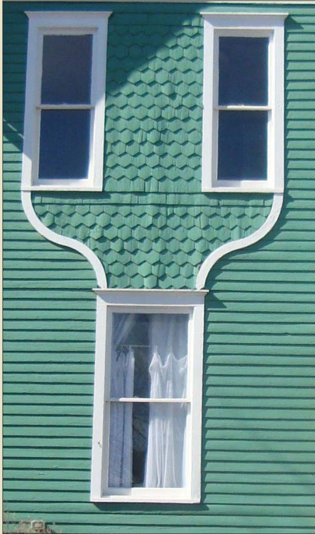
Retain and repair original windows, window surrounds and screens using materials that match the original.
