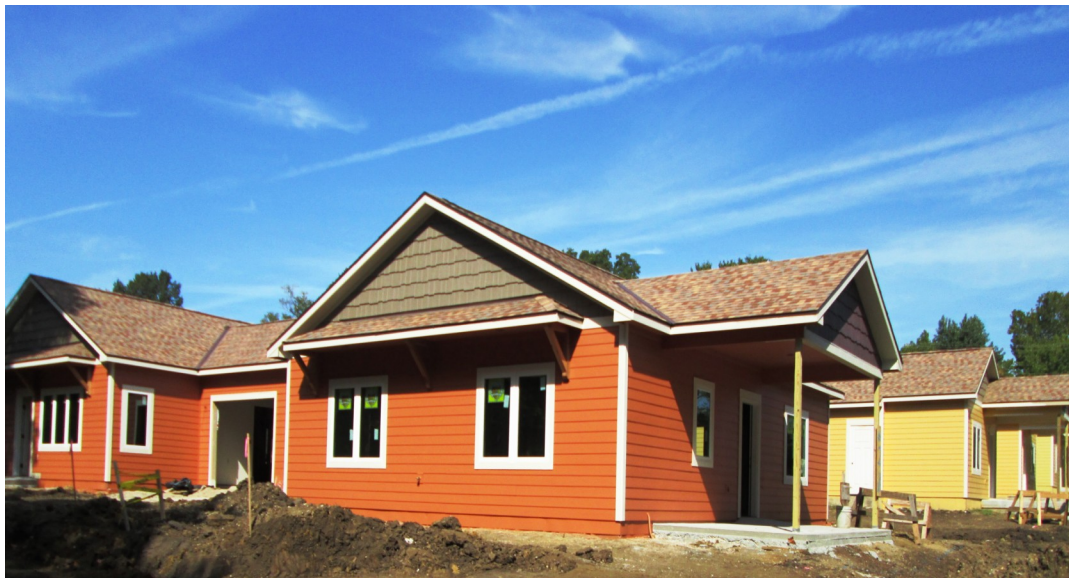
Exterior finishing of the same framed cottages on the 2500 Cedarwood.
