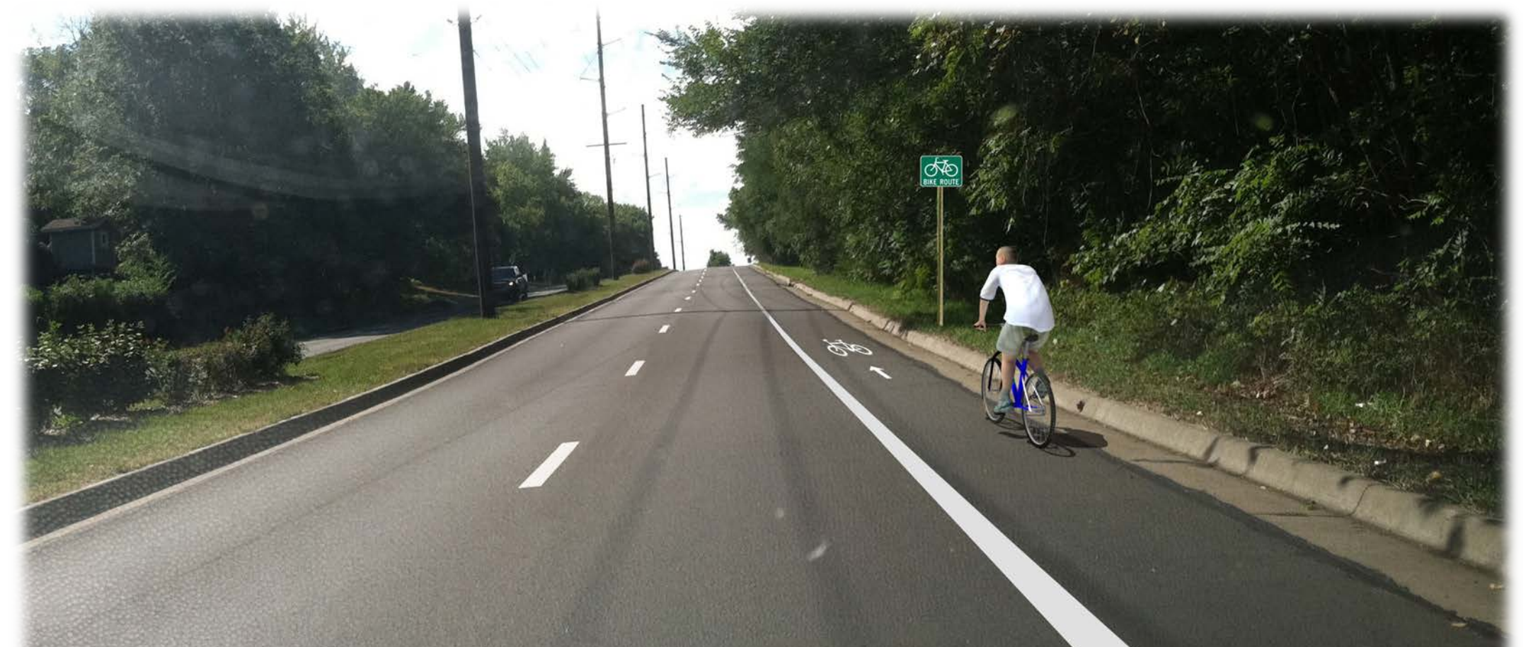
Kasold Drive in Lawrence (example of a marked bicycle climbing lane)
