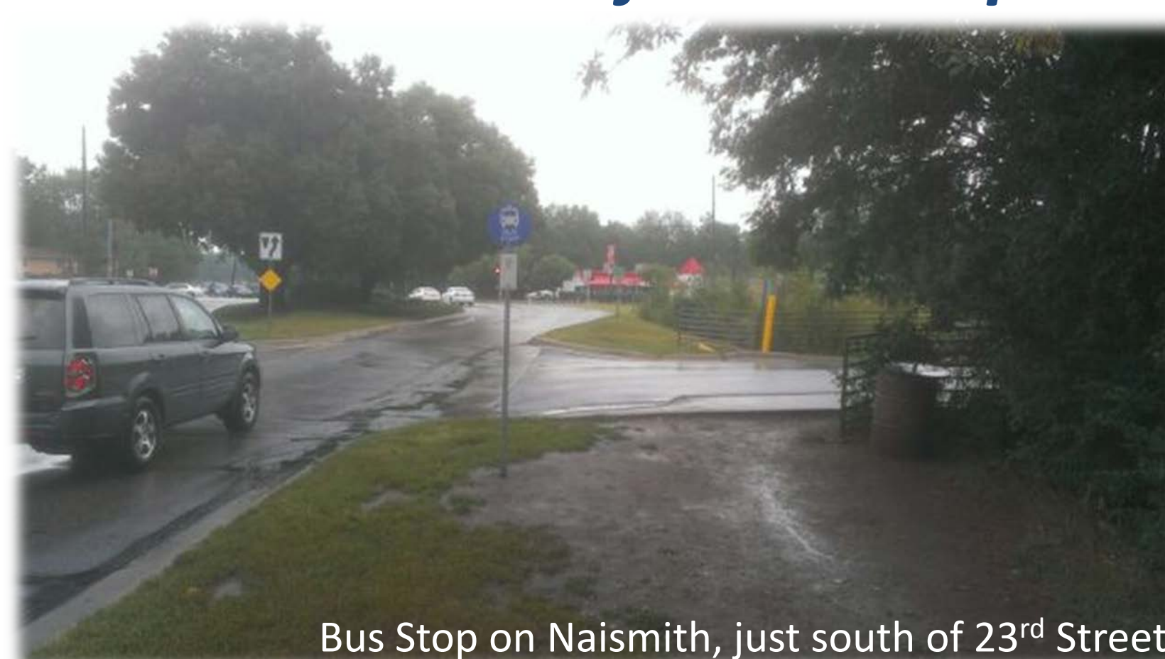
Lack of Concrete Pads and Shelters at Major Bus Stops
