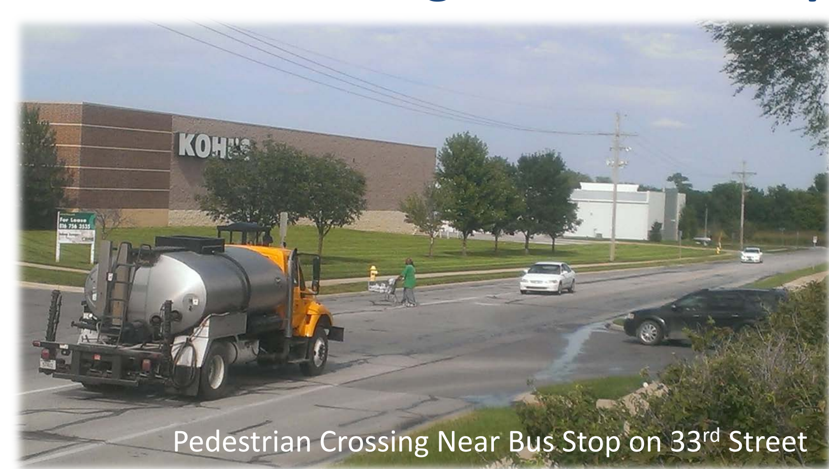
Pedestrian Crossings Near Bus Stops
