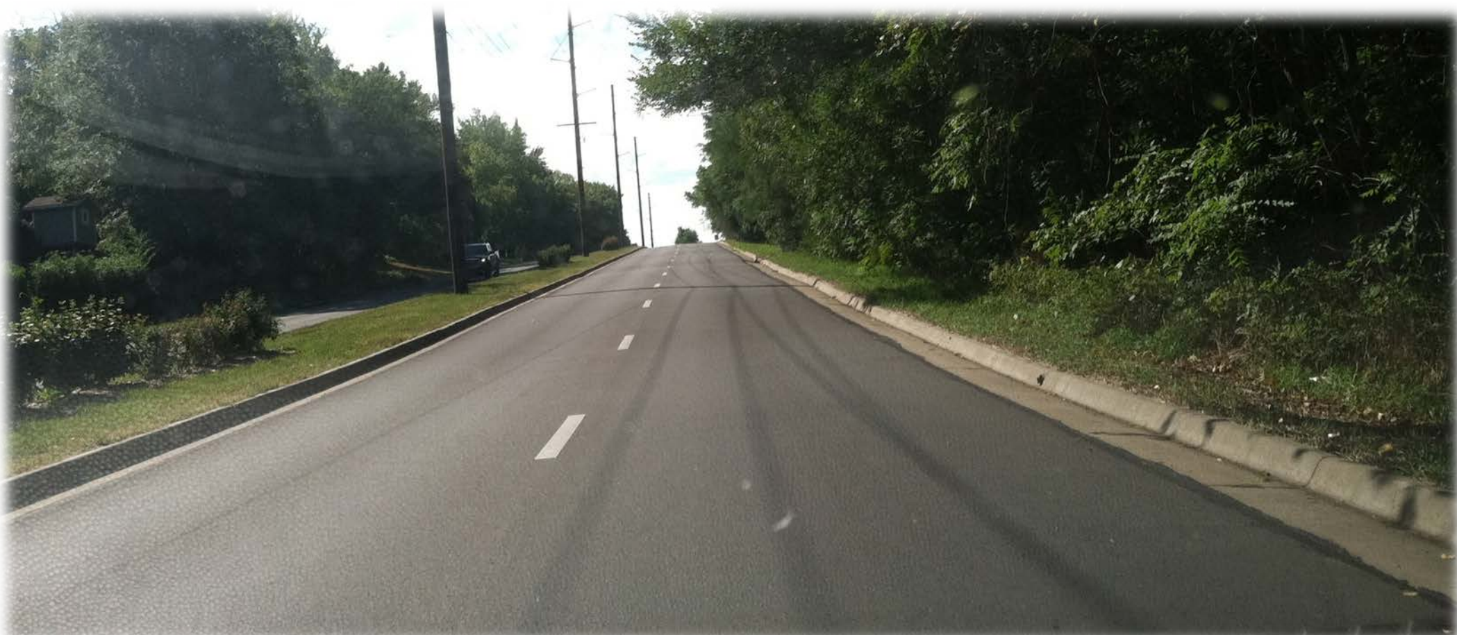
Kasold Drive in Lawrence (example of a marked bicycle climbing lane)
