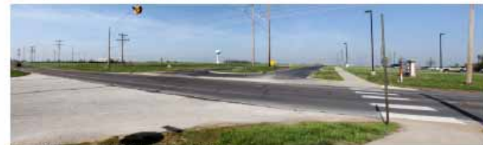
Figure 19. Crosswalk at E 2200 Road and 23 rd Street.
