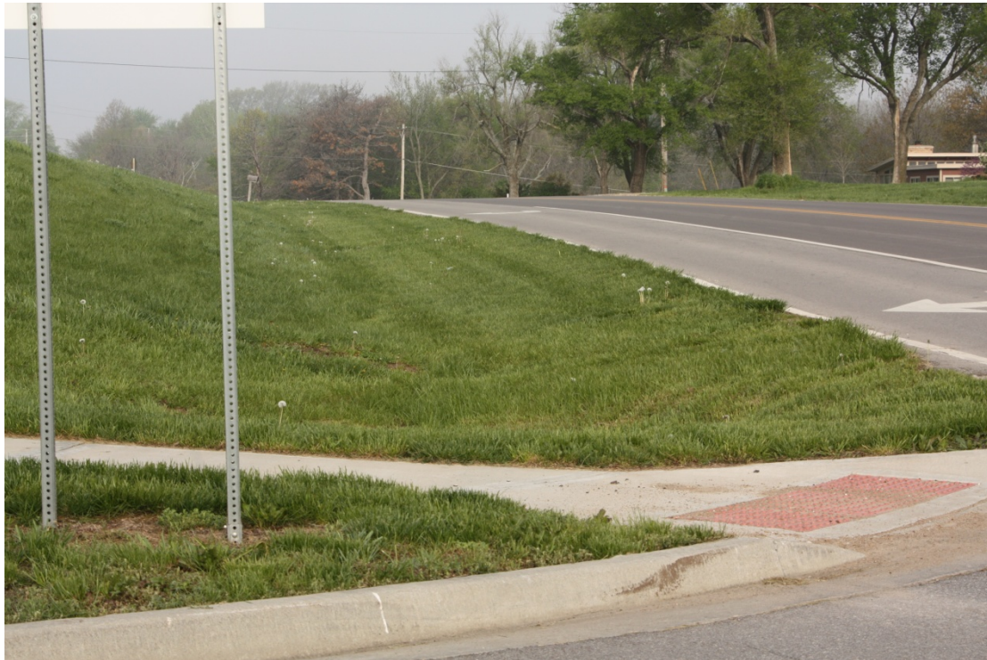
Figure 7. Sidewalk to the front door of the school dead-ends at N 1400 Road where there are no other sidewalks to tie into.
