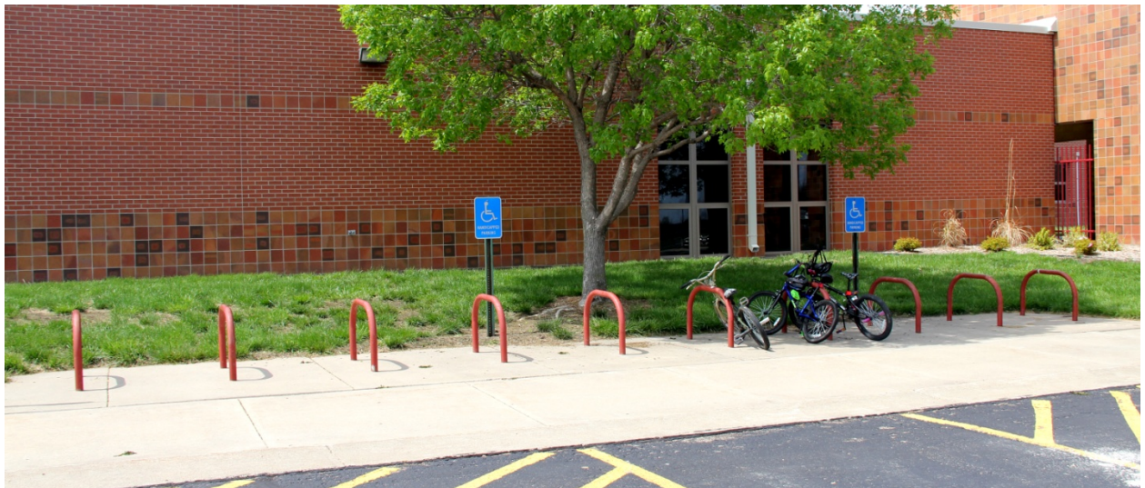
Figure 14. Half "H" style bike racks are provided on the east side of the school, next to the staff parking lot.
