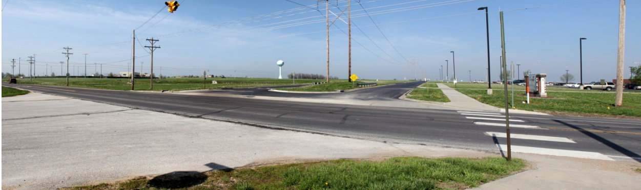
Figure 19. Crosswalk at E 2200 Road and 23 rd Street.
