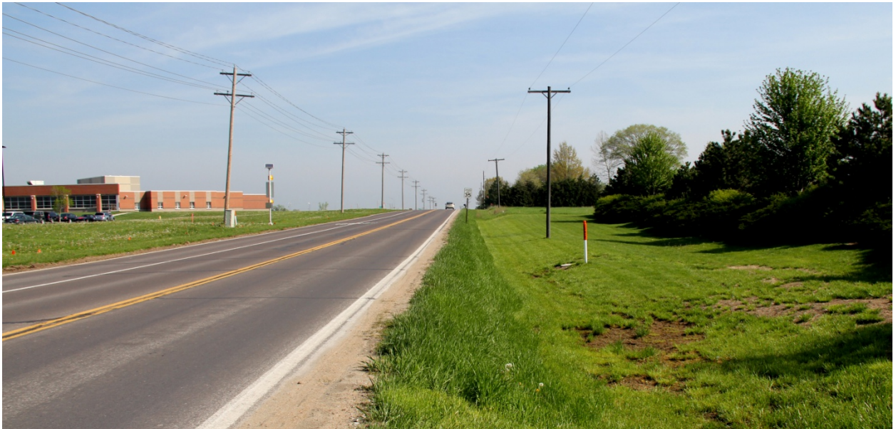
Figure 16. East 2200 Rd is a two lane road with no sidewalks and ditches on each side and is the only road connecting the Middle School to surrounding development.
