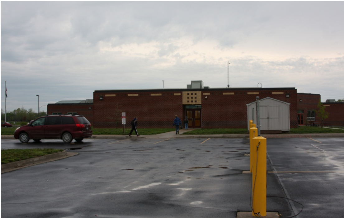
Figure 35. Baldwin City Intermediate School's south entrance accommodates walkers, bicyclists and students dropped off by car.
