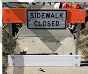
Pedestrian barricade placed across the entire pathway at location of closure
