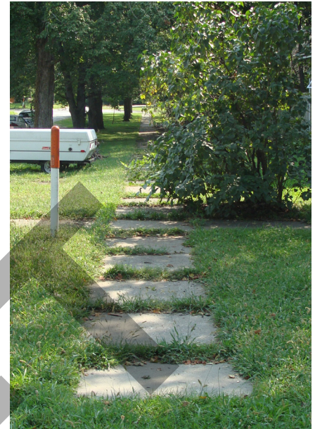
Figure 3-5: Sidewalk Defects
