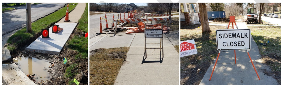
Figure 8: Incorrect Pedestrian Accommodations in Work Zones
