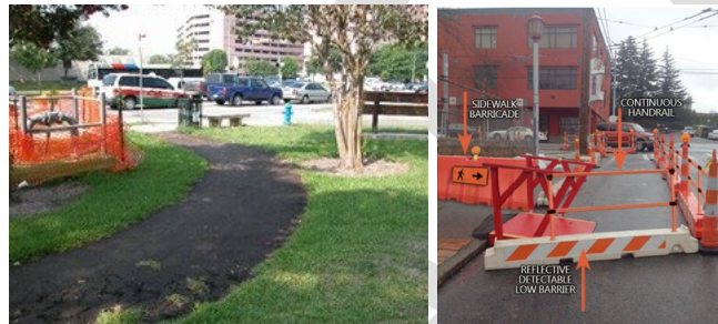
Figure 10: Appropriate Pedestrian Detours When No Opposite Sidewalk Option
