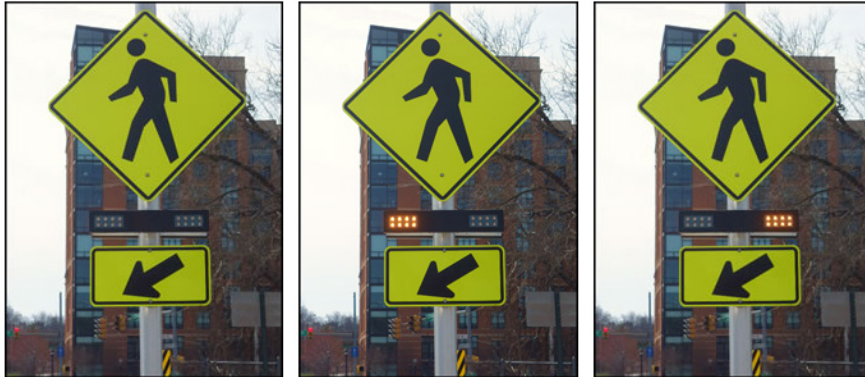
RECTANGULAR RAPID FLASHING BEACON SEQUENCE AT CROSSWALK. MUTCD.
