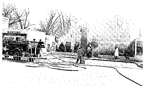
One of the many times the Southern Pit is on fire Number Two station does not have very far to go on this call, the Southern Pit is directly across the street from the station
