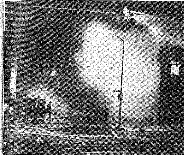
Lawrence firemen battle flames and chilling temperatures in the 20's at the Lawrence Launderers and Dry Cleaners commercial laundry facility. at 10th and New Hampshire, loss estimated over $200,000
