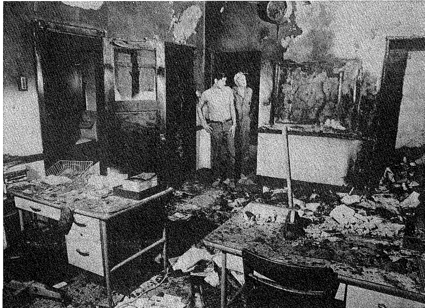
ARSONIST HITS SCHOOL — Above Bruce Nilsen, left and Merton Harmon, school district maintenance workers, examine damage to the office of the New York School
