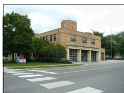
Station No. 1 746 Kentucky St. Lawrence, KS 66044
