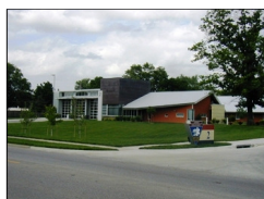
Station No. 2 2128 Harper St. Lawrence, KS 66046
