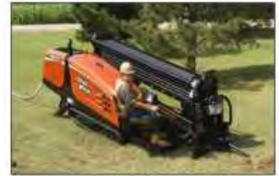
Horizontal Drilling Eliminates Trenches
