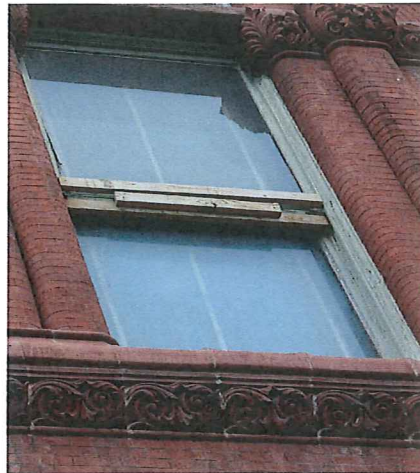
Window Detail: temporary sash repair
