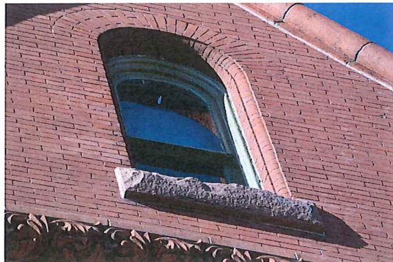
Restored Attic Window, east facade
