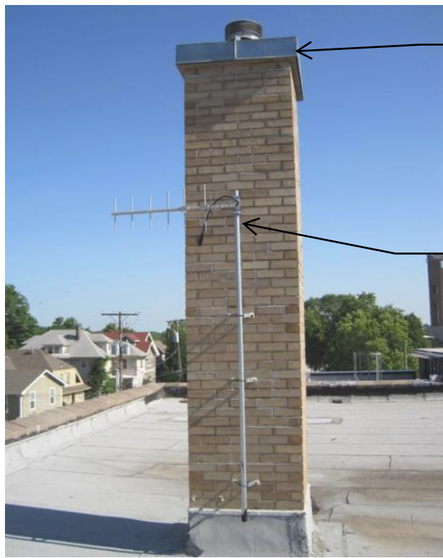
1 SOUTH FACE OF CHIMNEY PHOTO
