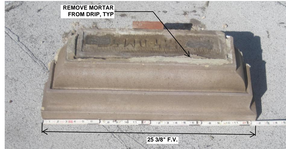
2 BOTTOM OF PILASTER NOSING PHOTO
