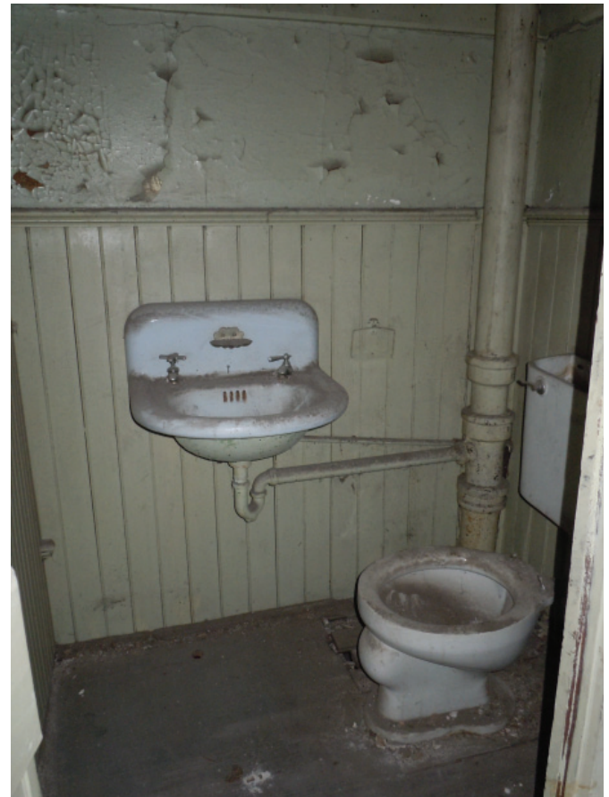
Second Floor Toilet
