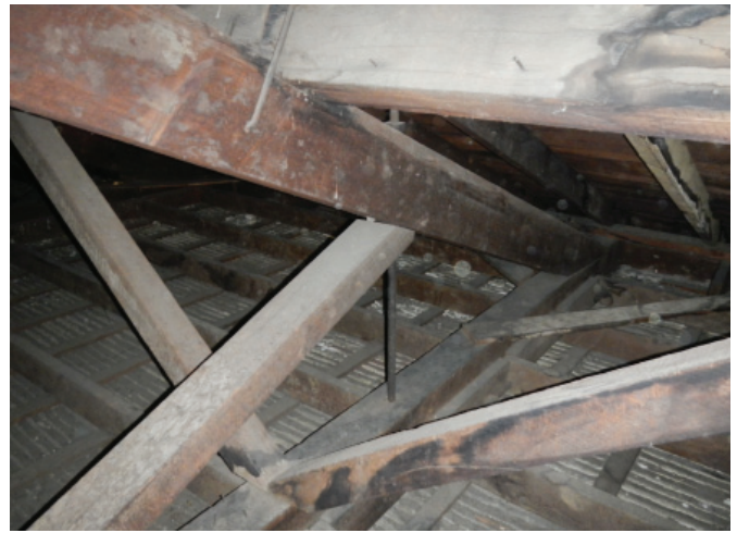
Heavy Timber Roof Truss
