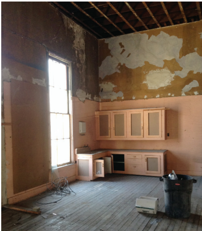
First Floor Kitchenette
