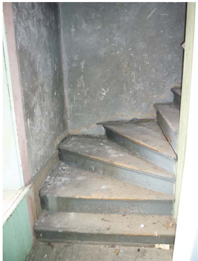
The staircases and tin ceilings are considered Class "B" features.
