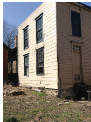
Discharge of the Exhaust Fan for First Floor Ventilation Hood – Located in Window on South Side of Building
