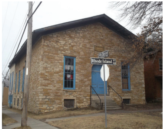
Turnhalle Looking Southeast
