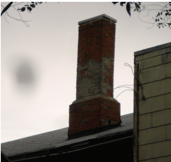
Chimney on South Slope of Roof
