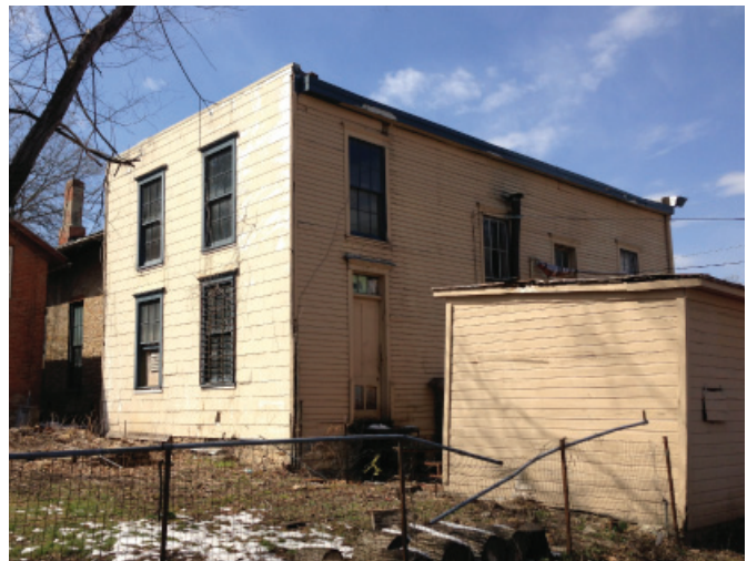
Turnhalle Looking Northwest
