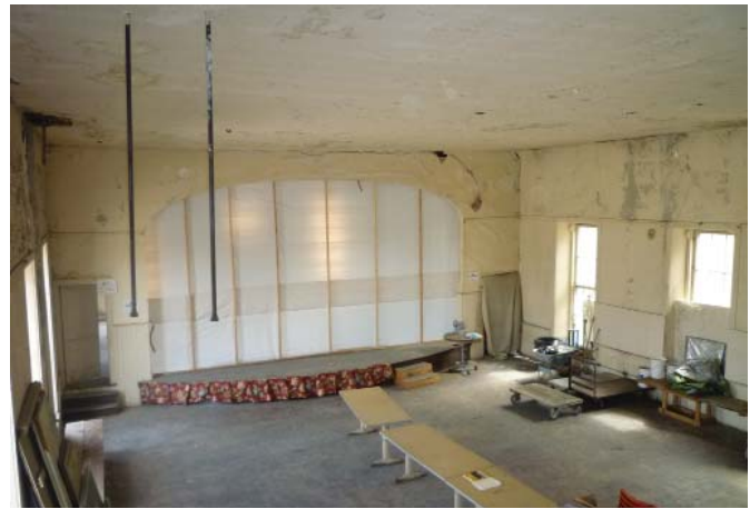
While the Main Hall exhibits minimal detailing, the architectural features that do exist are significant and help define this highly significant space. As such, the wood wainscot, window and door surrounds (woodwork), plasterwork and wood floors should be retained and restored, as well as the open space of the main hall.
