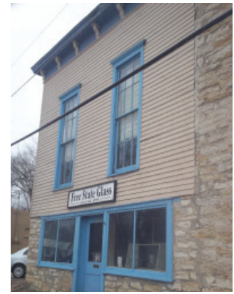
Original Bracketed Eave and Wood Siding on North Elevation
