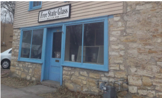
Basement Entrance Doors on North Elevation
