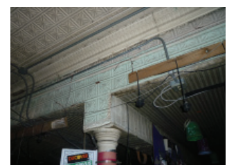
Tin Wrapped and Bead-Board Wrapped Beams in Basement
