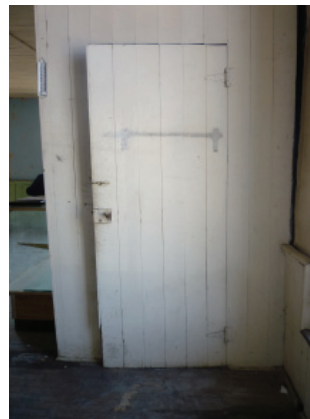
Board-and-Batten Door at Stair No. 1 to Basement and Original Hardware
