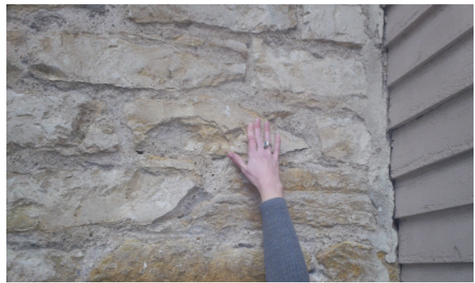
Original Pointing Mortar on South Elevation
