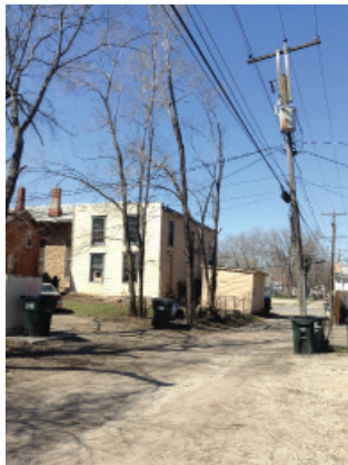
Main Electrical Transformer
