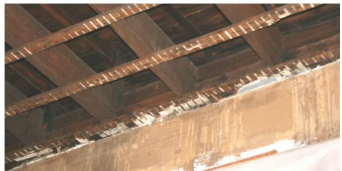
Connection between 2x12 Joists and Ledger
