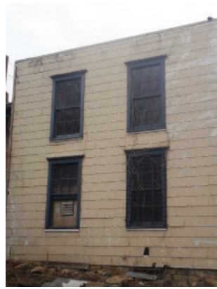
Cement Siding on South Elevation
