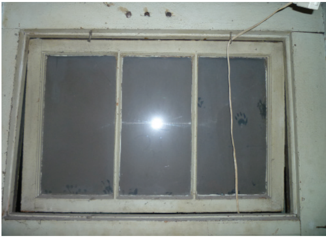
Interior Awning Sash of Basement Window
