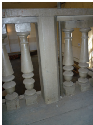
Detail of Balcony Balustrade. The balustrade is original due to the penetration of the tie rods.
