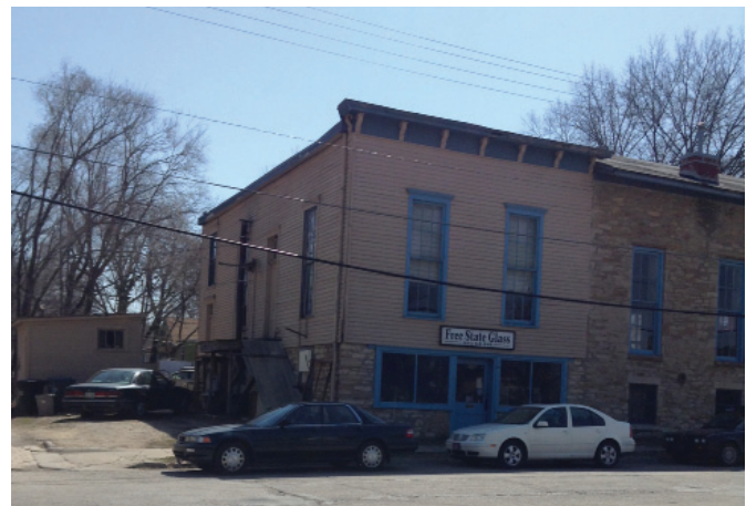
Gutter and Downspout for East Roof
