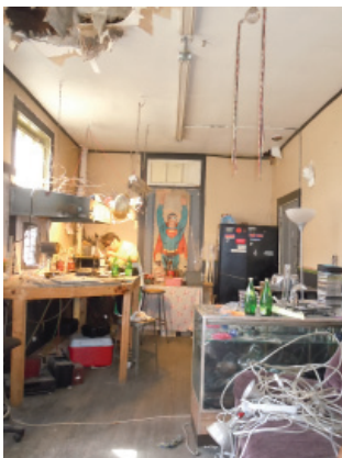
First Floor Ventilation Hood
