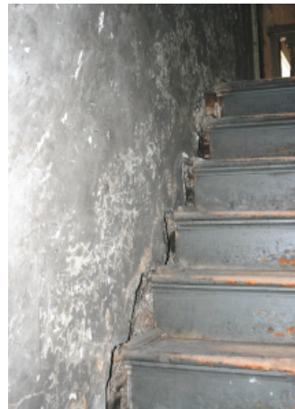
Northwest Stair between Lower Level and First Floor.
