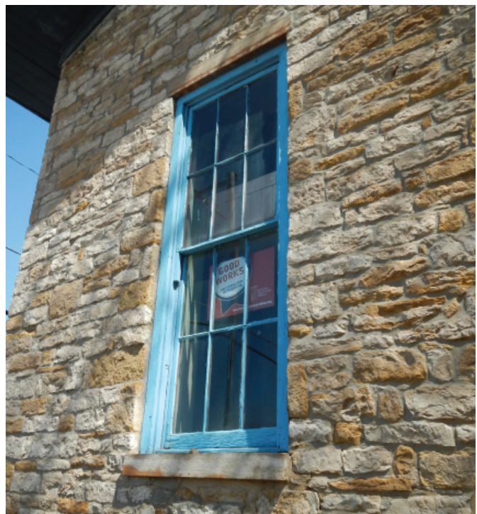
Original Wood Window on West Elevation
