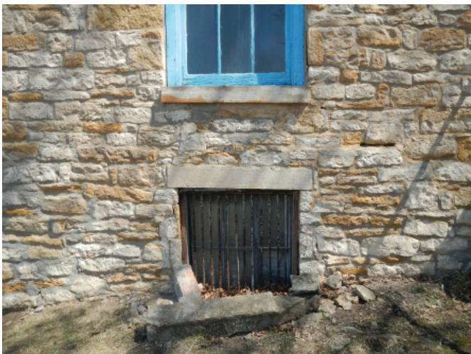
Typical Stone Construction Surrounding Basement and First Floor Windows
