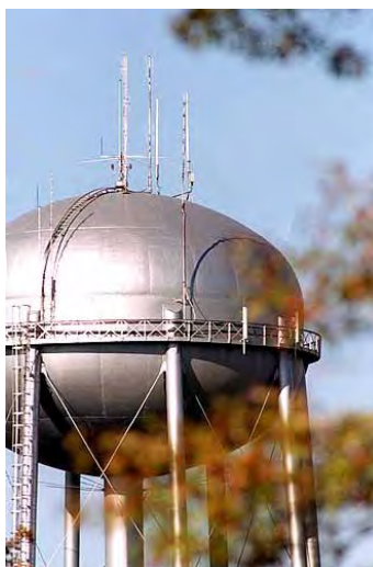
Stratford Water Tower Lawrence, Kansas
