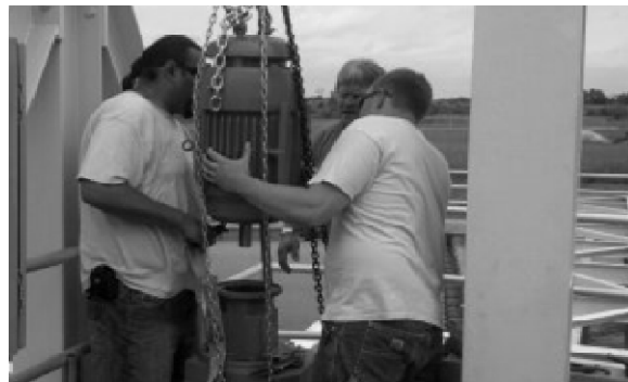
Maintenance replaces a worn pump on a basin at the Clinton Water Treatment Plant.
