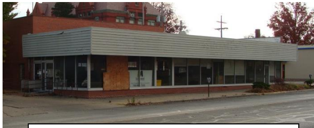
1040 Vermont Street Before Renovation
