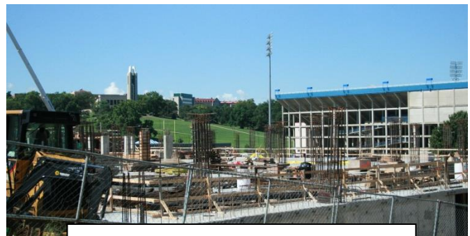
Project Under Construction
