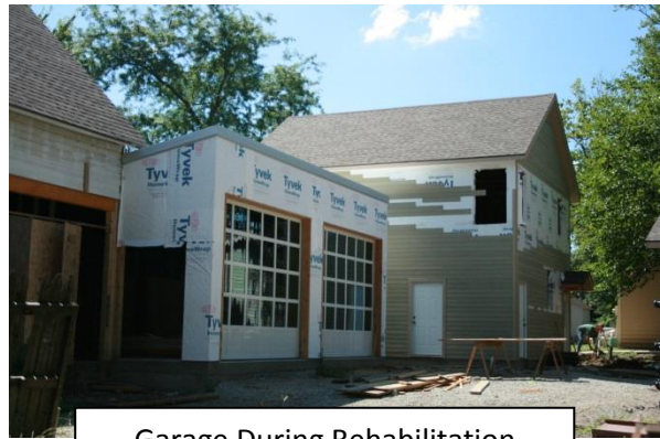
Garage During Rehabilitation
