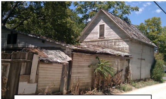
Barn Before Rehabilitation
