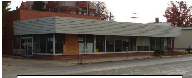
1040 Vermont Street Before Renovation
