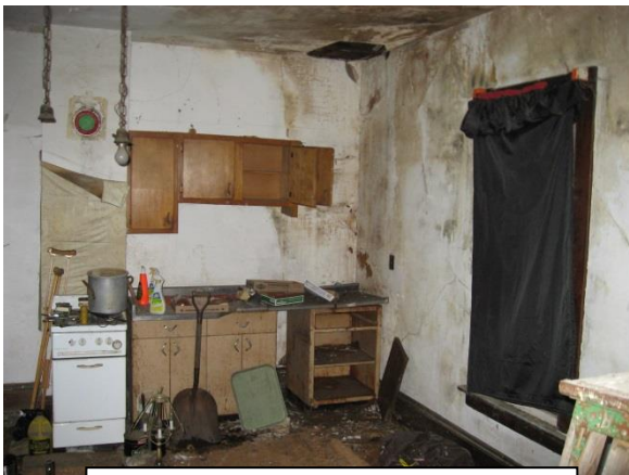
Kitchen Before Rehabilitation
