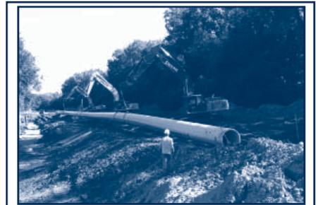
A new transmission line was recently installed 65-feet under the Kansas River to north Lawrence. The line increases reliability & system capacity.
