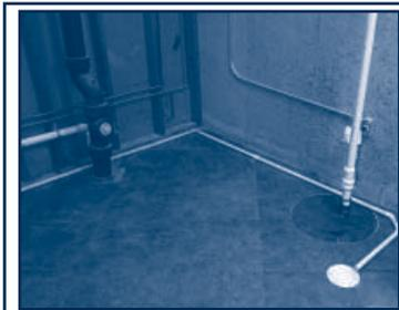
The EcoFlow Rapid Rain Water Reduction Program works with homeowners to repair identified areas where water is getting into the sewer system. Here, a sump pump is correctly redirected to discharge water to the outside, not into the city's sewer system.
