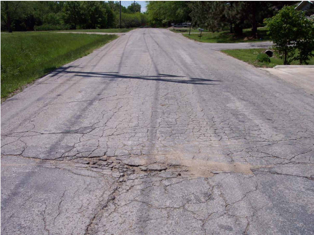
Iowa St south of Princeton Blvd (Residential, PCI = 29)
