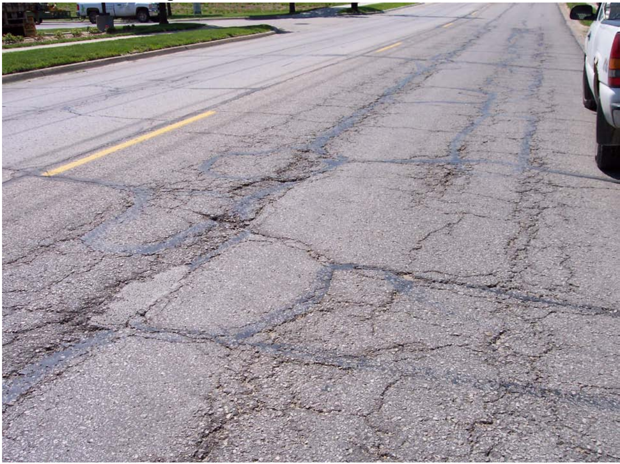
Iowa St, Kingston Dr to Princeton Blvd (Arterial, PCI = 47.6)
