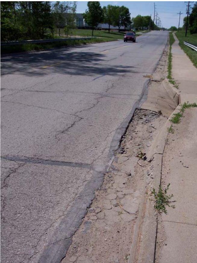
N Iowa St, Peterson Rd to Kresge Rd (Arterial, PCI = 58.95)
