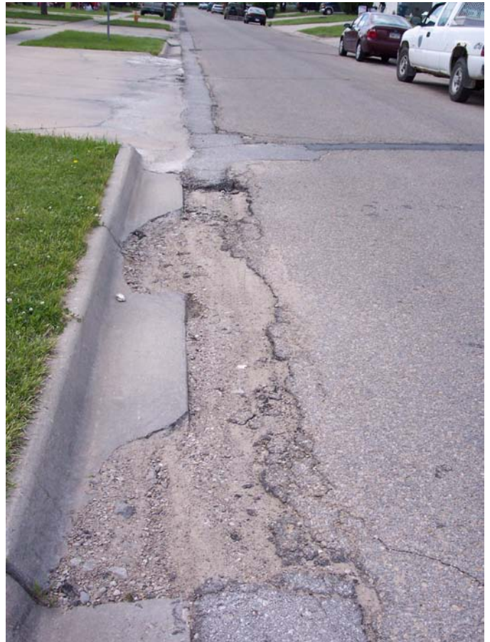
Overland Dr, Monterey Way to Eldridge St (Residential, PCI = 52.3)
