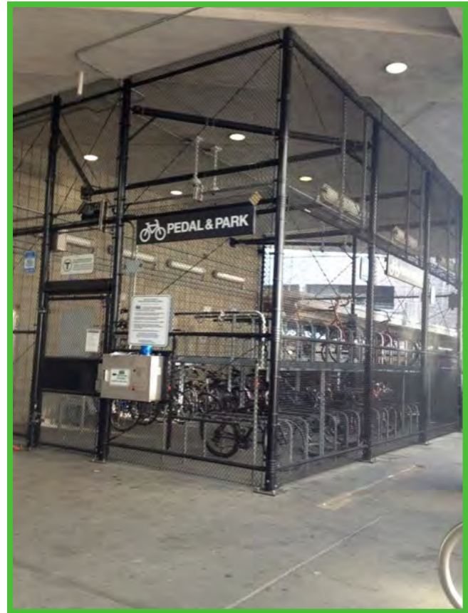
Example of large scale bicycle parking in Boston. Variations of this bicycle storage could be incorporated throughout Lawrence to support the development of a truly multimodal transportation system.
