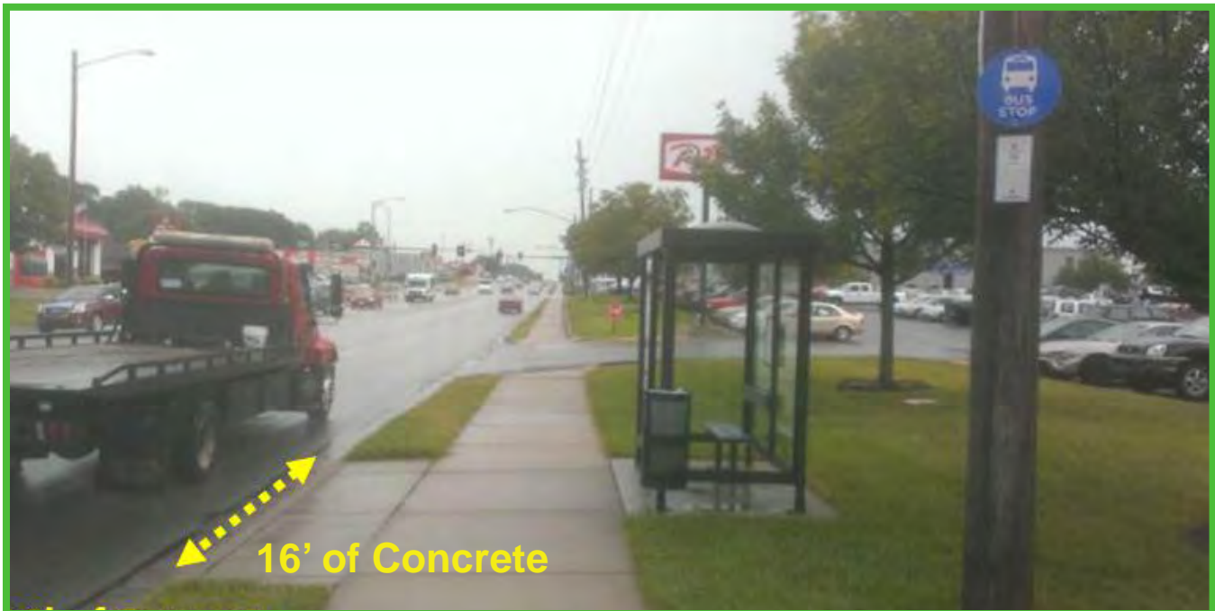
Figure 5-7: Example of Wide Concrete Boarding Area
