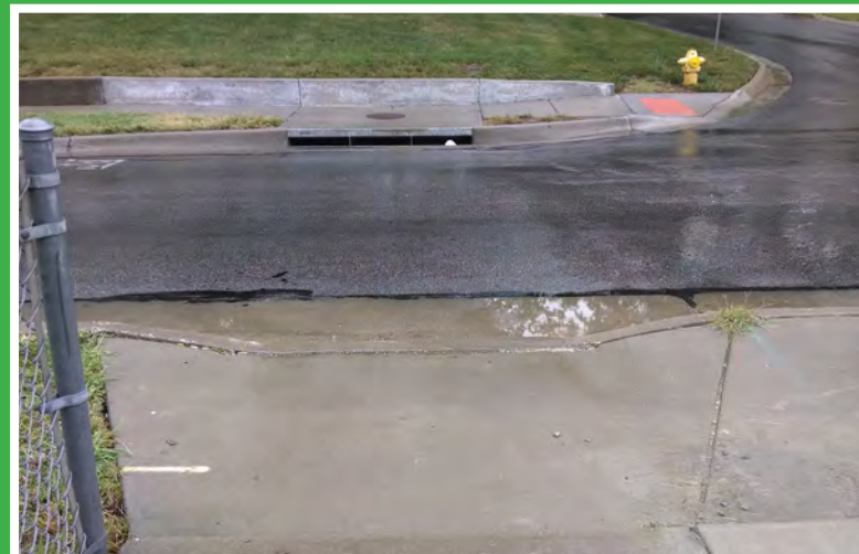
Figure 5-16: (Below) Naismith Drive – Curb Ramp Accessibility Issues.
