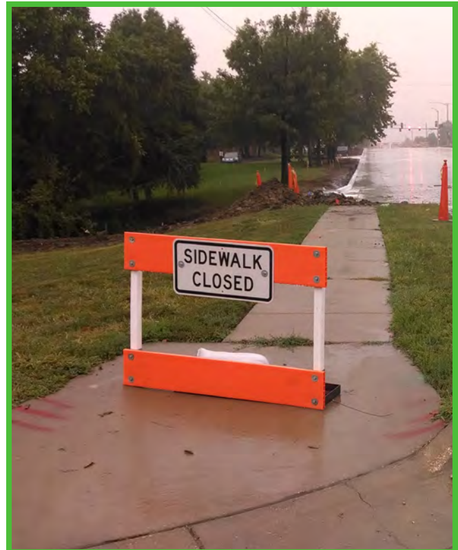
Wakarusa sidewalk being installed as part of roadway improvements
