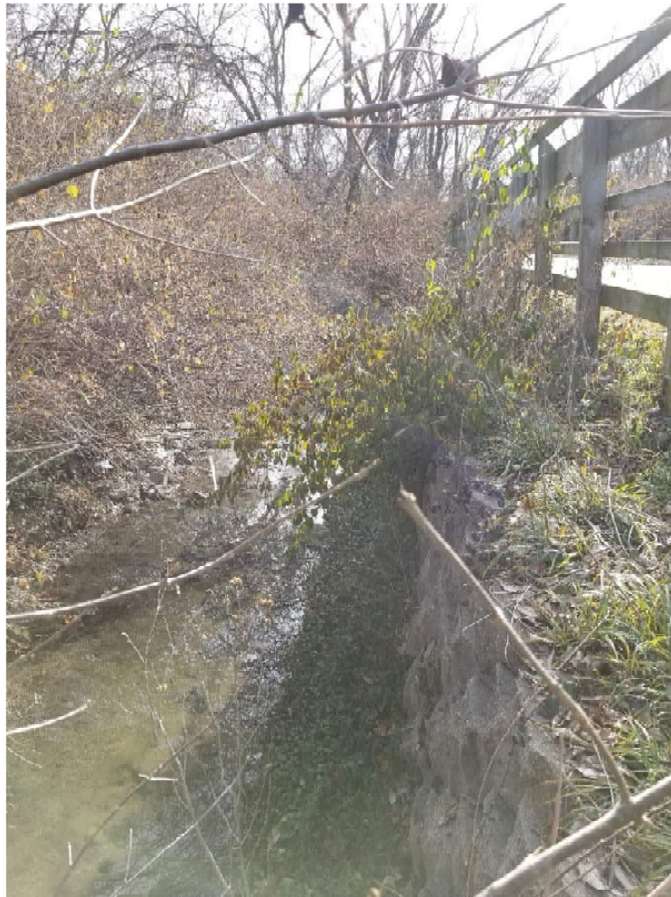
Figure 6 – Photo of Pavestone Wall, Looking South Along Fence, Trail
