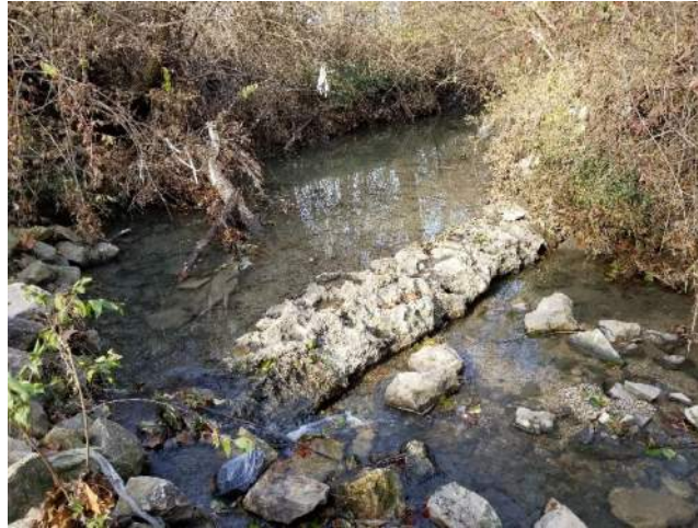
Figure 7 – Photo of Sanitary Encasement Looking Upstream, North
