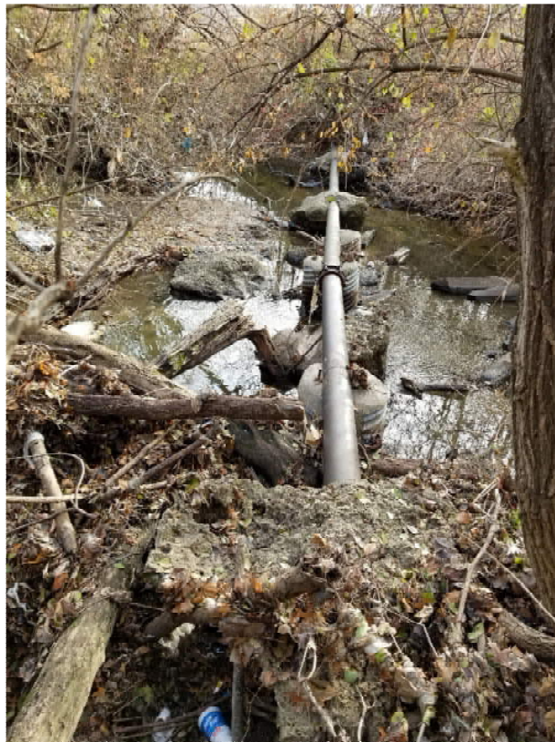
Figure 13 – Photo of Waterline Crossing, Possibly Abandoned, Not on City Mapping, Looking Southeast
