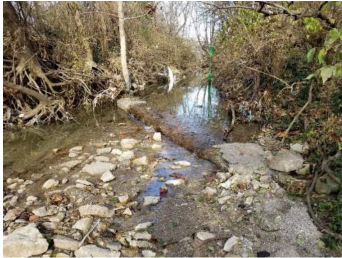
Figure 4 – Photo Looking Upstream, North at Sanitary Encased Crossing
