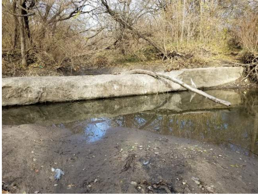
Figure 12 – Photo Looking Upstream At large Encasement, North
