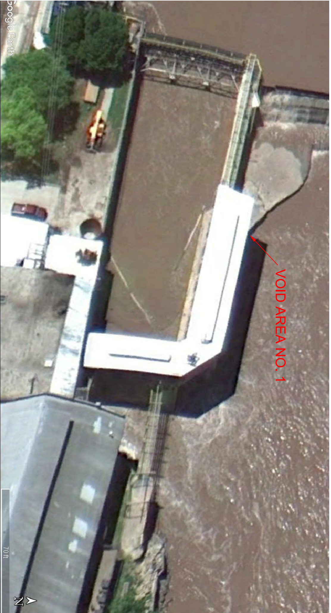
VOID AREAS - SOUTH DAM AREA
