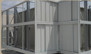
Installation of screen around unit with pipe-chase.
