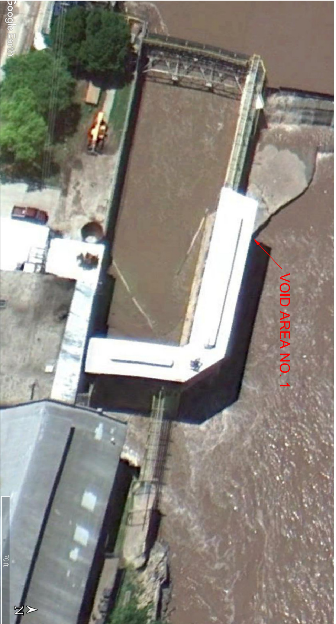
VOID AREAS - SOUTH DAM AREA
