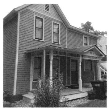
Additions flush with the side of the existing house have been built in the area for decades. The separation of the original from the new by a vertical trim board is quite common.
