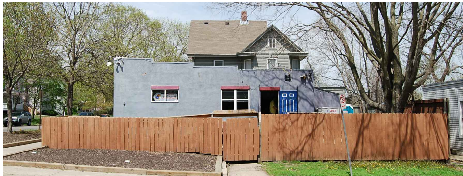
5 SOUTH ELEVATION BEFORE RENOVATION SCALE: 1/8" = 1'-0"
