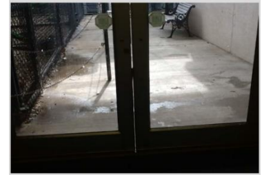
Gap Between Doors Due to Worn Weather Stripping at Prairie Park Nature Center
