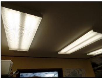
Existing Solid Waste T8 Lighting
