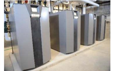
Modern Condensing Boiler With Higher turndown
