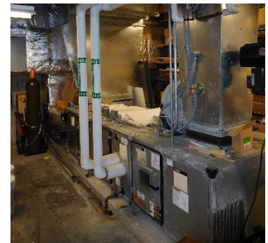
Single Zone Constant Volume Air Handling Unit
