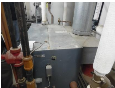
Existing Heating Water Boiler
