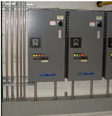
Variable Speed Drives for Pumps
