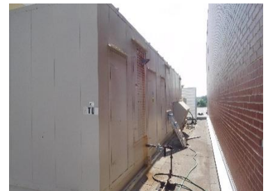
Existing Packaged Dehumidification Unit
