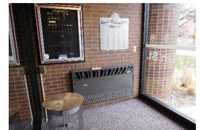
Electric Cabinet Heater at Main Entry
