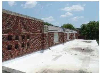
Rubber Membrane Roof
