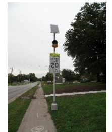
Solar-Powered School Beacon Uses No Utility Electrical Power
