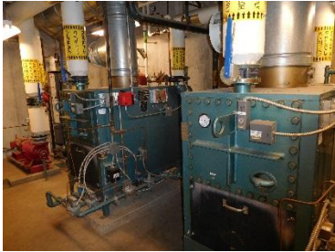
Existing Atmospheric Boilers
