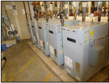
Existing building boilers
