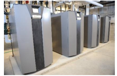
Condensing Boiler Plant
