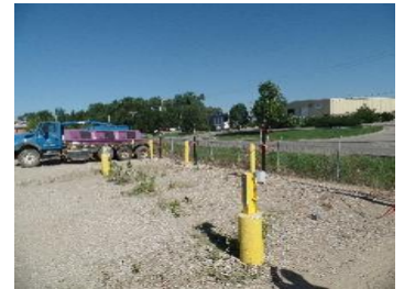
Block Heater Receptacles on Bollards
