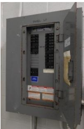
Panelboard with Corrosion
