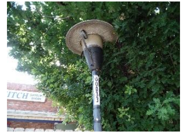
Aged and Distressed Pole To Be Replaced
