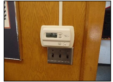
Existing Stand-Alone, Non-Programmable Thermostat
