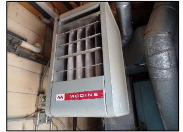
Gas-fired unit heater
