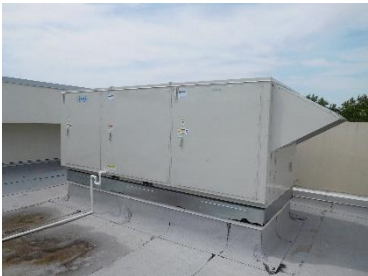
Typical VAV Rooftop Unit
