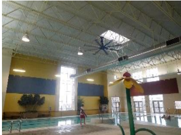
Existing Supply Ductwork in Leisure Pool
