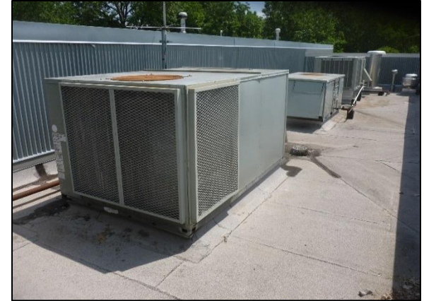
Outdated RTU at Fire Station No. 2
