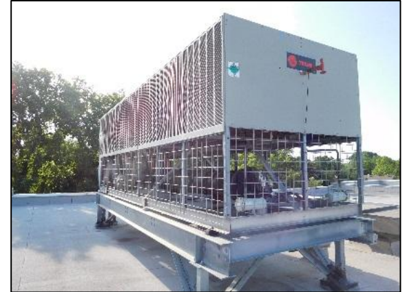
Existing LAC air-cooled chiller
