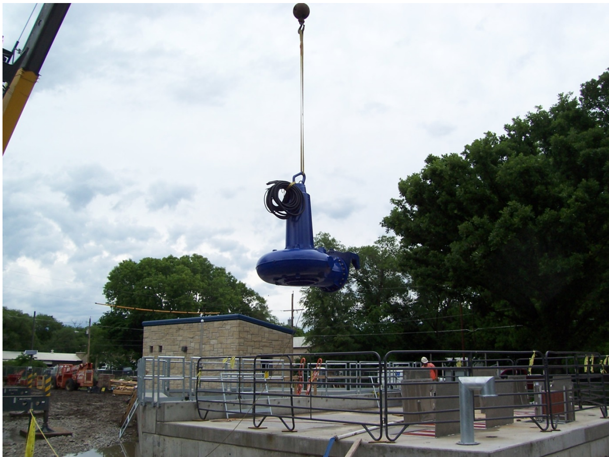
New pump at pump station
