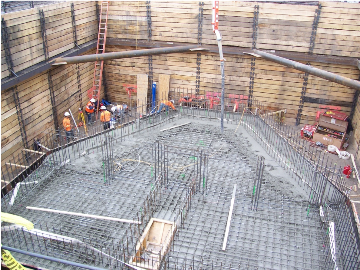
Concrete Placement of New Pump Station
