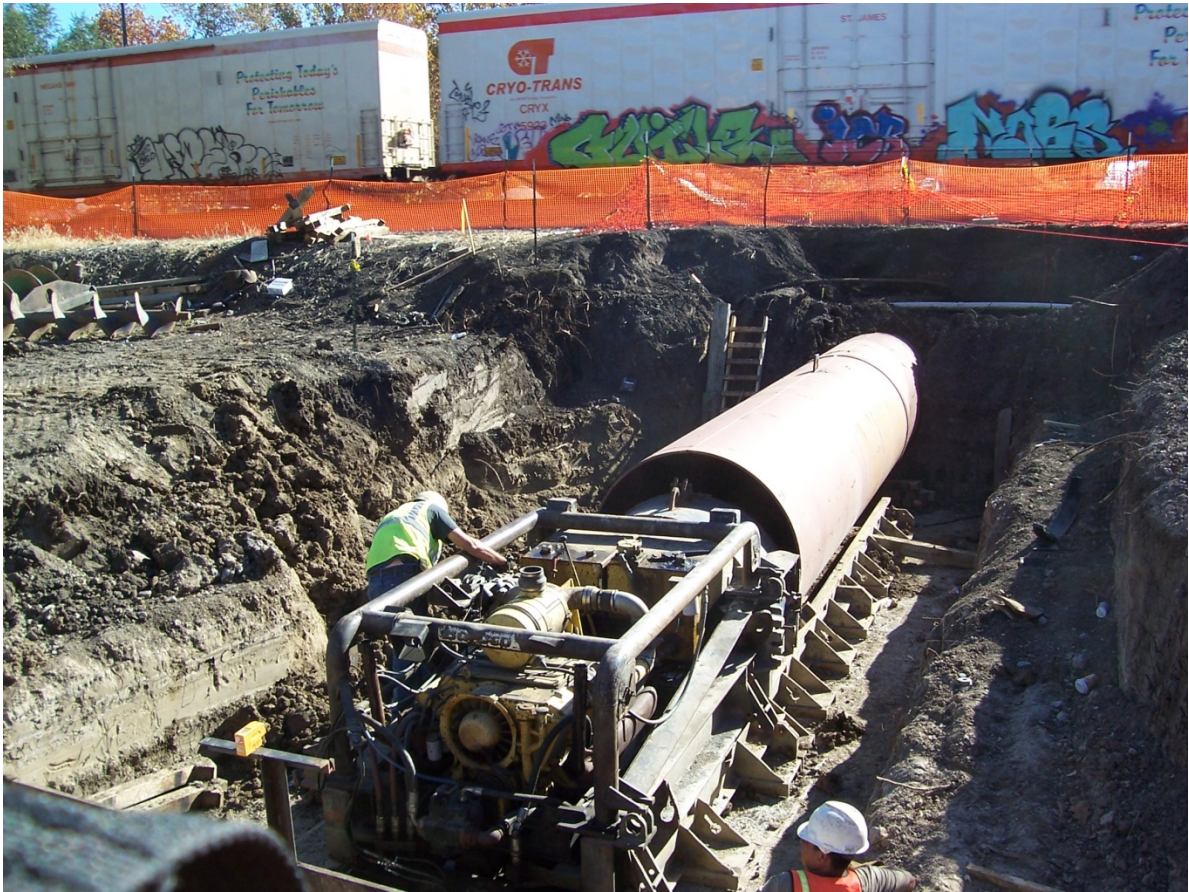
Boring under the Union Pacific Railroad Tracks
