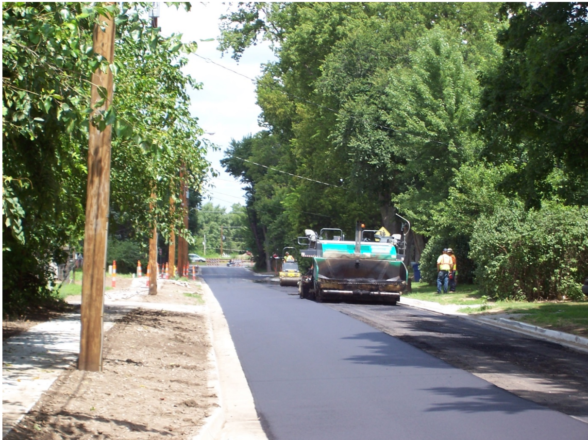
Surface lift of asphalt on 6 th Street
