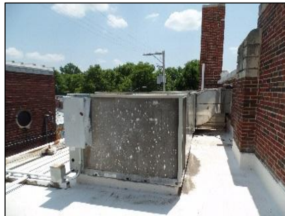
Hail Damage on RTU
