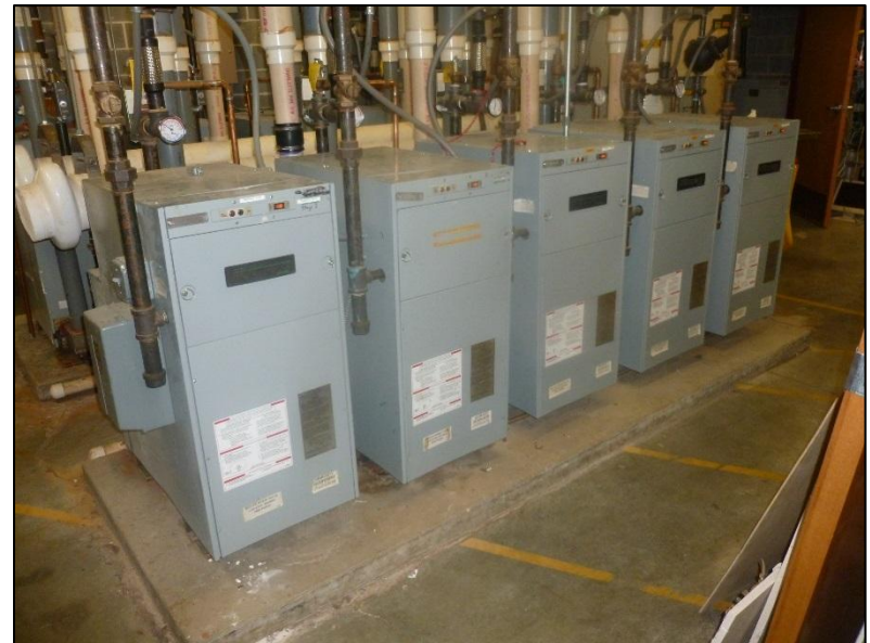
Existing 20-year-old condensing boilers
