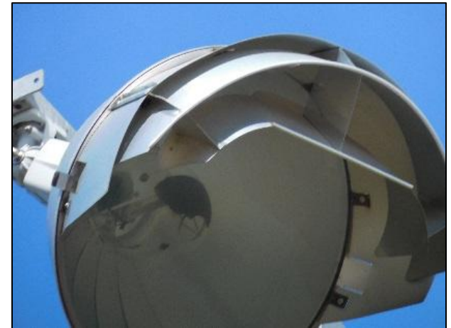
Existing metal halide lighting
