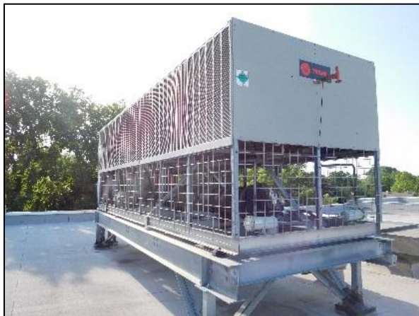
Existing air-cooled chiller
