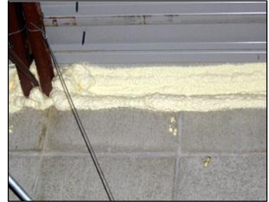
Sealing between wall and roof
