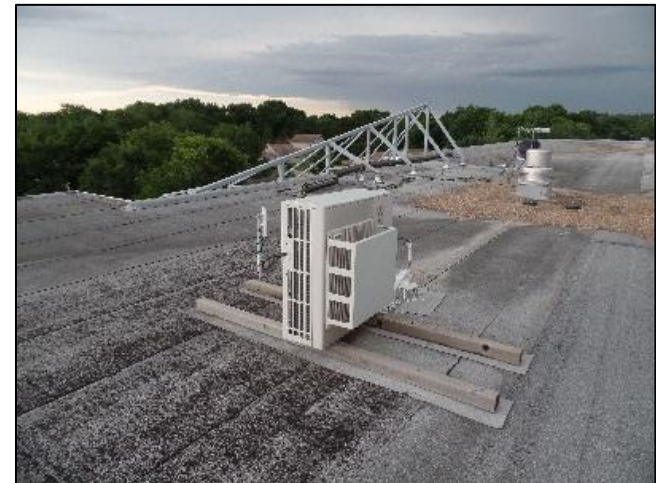
Substantial de-mineralization on roof
