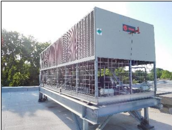
Existing air-cooled chiller
