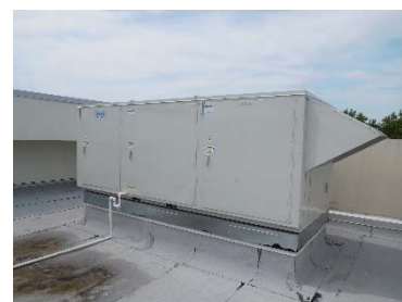
Typical VAV Rooftop Unit
