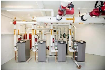
Example High Efficiency Hot Water Plant
