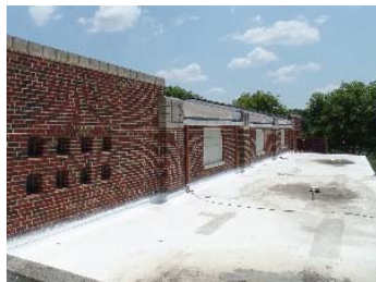
Rubber Membrane Roof
