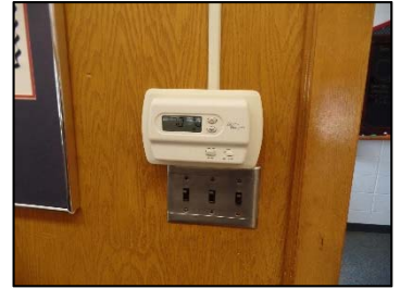
Existing Stand-Alone, Non-Programmable Thermostat
