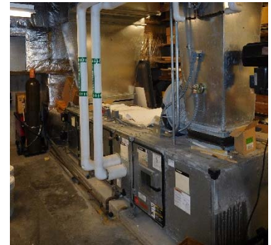
Single Zone Constant Volume Air Handling Unit
