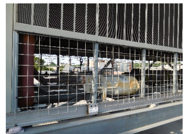
Existing Helical Rotary Screw Compressor
