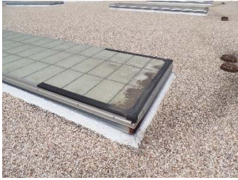
Failing Skylight
