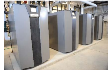
Condensing Boiler Plant
