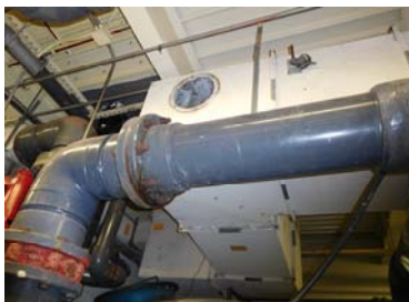
Decommissioned Exhaust Duct
