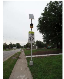
Solar-Powered School Beacon Uses No Utility Electrical Power
