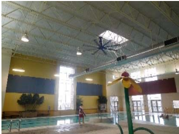
Existing Supply Ductwork in Leisure Pool
