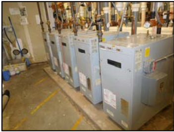
Existing building boilers
