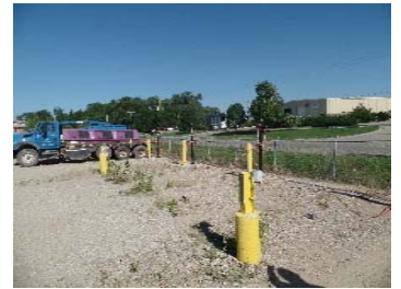
Block Heater Receptacles on Bollards
