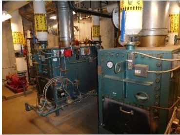
Existing Atmospheric Boilers
