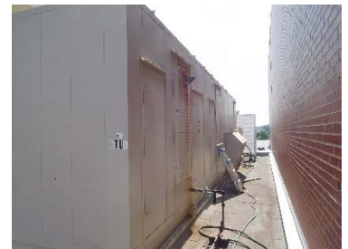
Existing Packaged Dehumidification Unit
