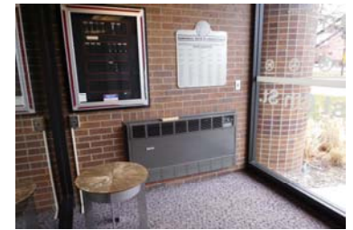
Electric Cabinet Heater at Main Entry
