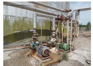
Twin 50HP Pump Motors at a Venture Park Holding Tank
