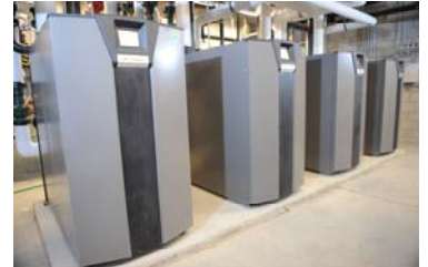
Modern Condensing Boiler With Higher turndown
