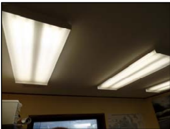
Existing Solid Waste T8 Lighting
