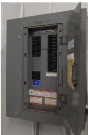
Panelboard with Corrosion
