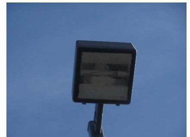
Shoebox Style Light on a Tall Pole
