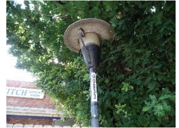
Aged and Distressed Pole To Be Replaced
