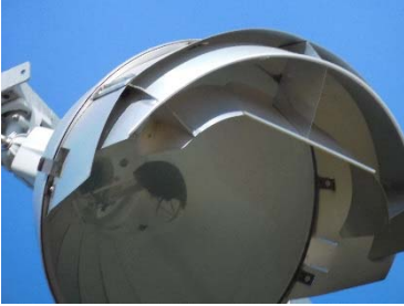
1000W Metal Halide Lamp at Outdoor Tennis Court
