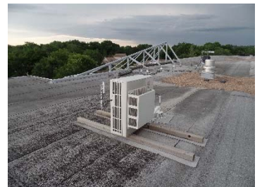
Substantial De-Mineralization on Community Health Building Roof
