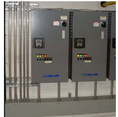
Variable Speed Drives for Pumps
