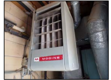
Gas-fired unit heater
